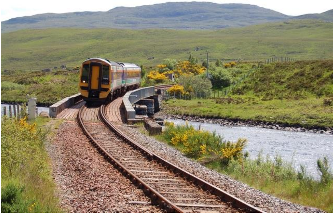
Figure 2.2 A single track railway in UK [10]
