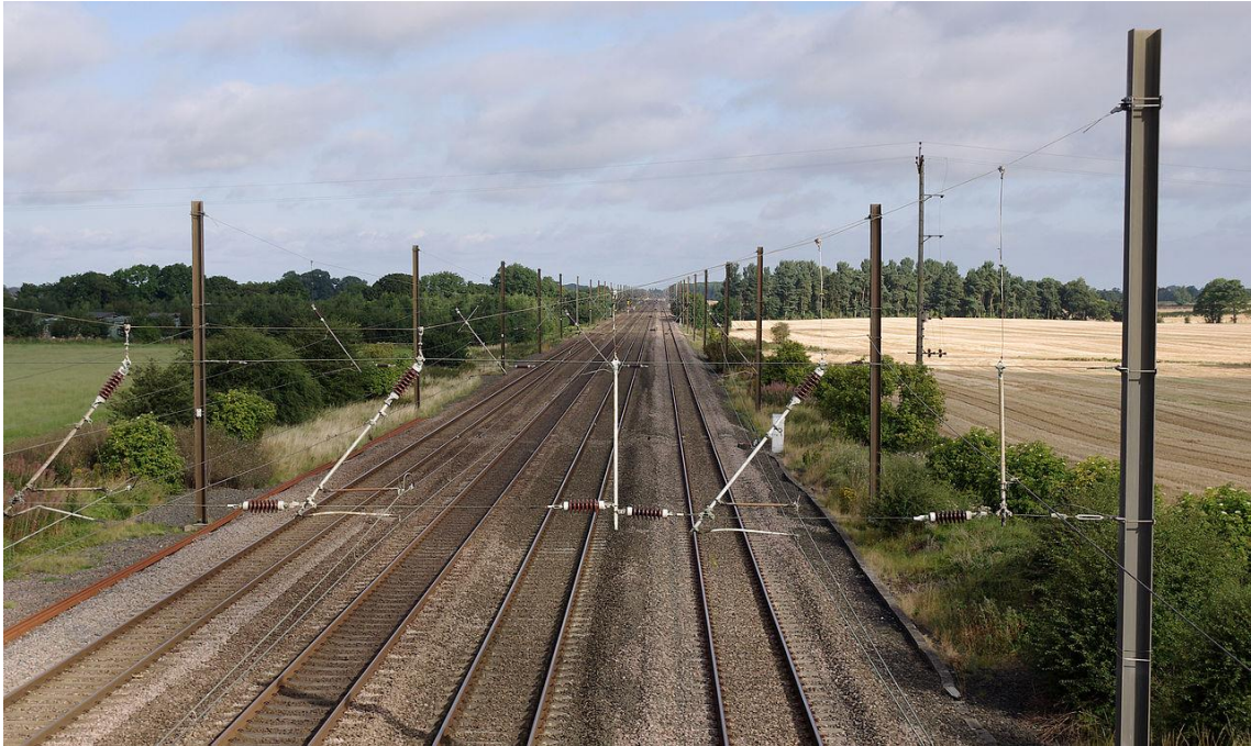
Figure 2.4 A multiple track line from UK [12]
