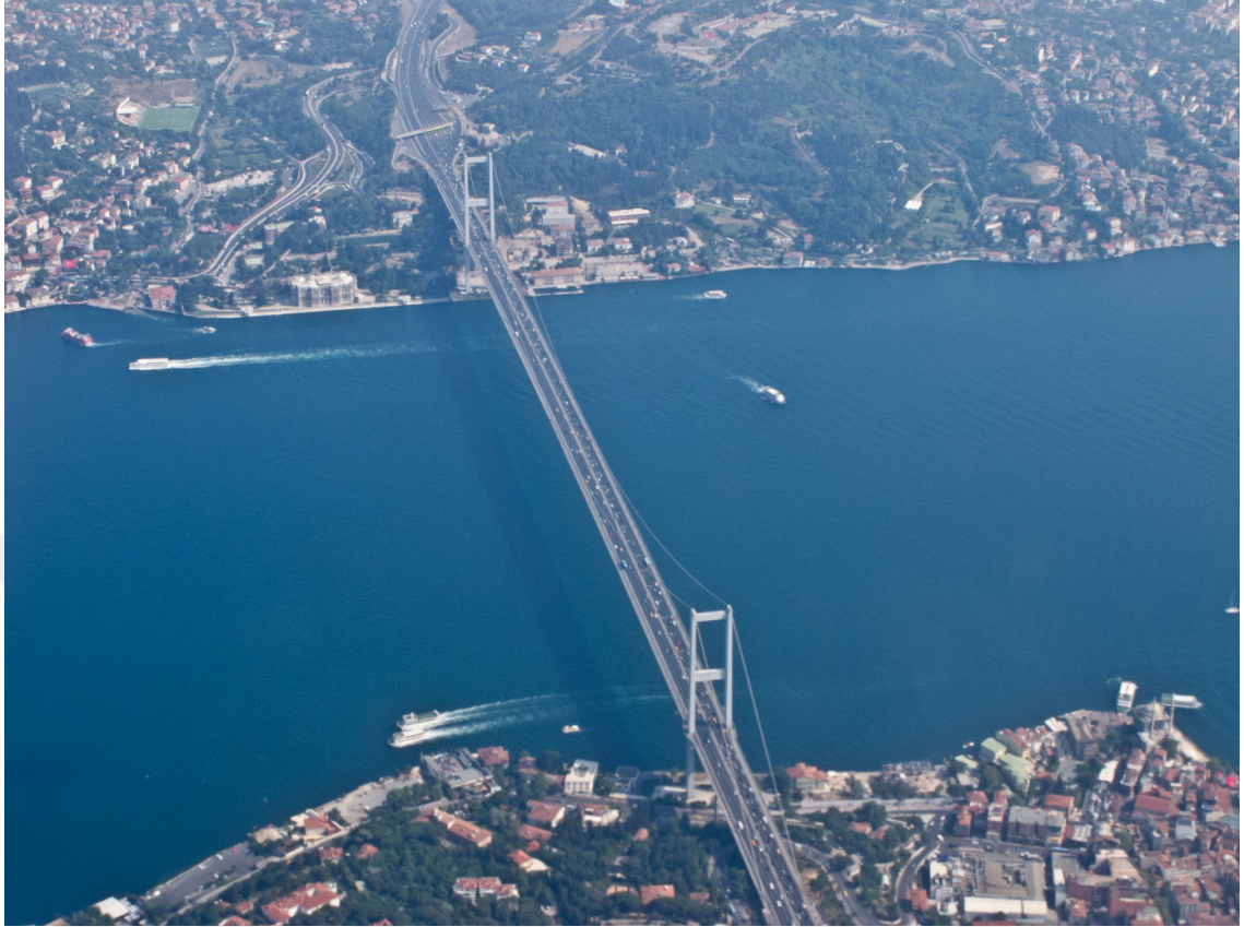
Figure 2.3 The view of the Bosphorus Bridge from above[16]
