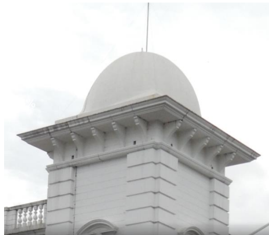
3. Overhanging square- based with support brackets
