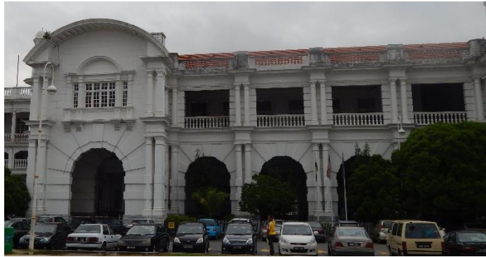
Figure 4.97 Voussoir arches dominating the ground floor creating arcades in Ipoh station building
