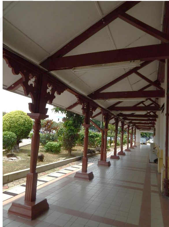
2. Wooden column with decorative spandrels,
