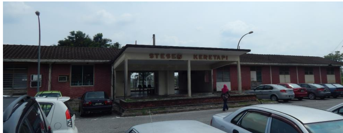
4. Facade view of the station building.
