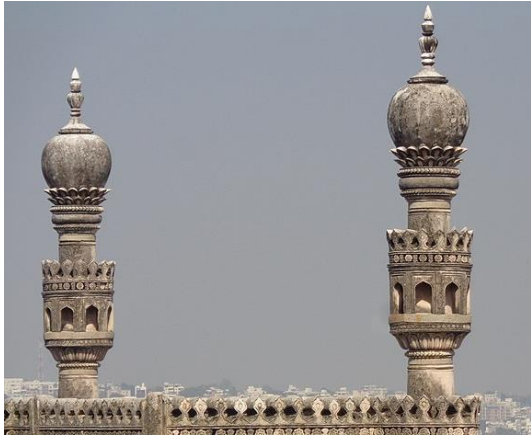
Figure 4.78 The lotus flower resembling finial built around 1600s, the oldest example known is seen in Mosque of Ibrahim, India [151]
