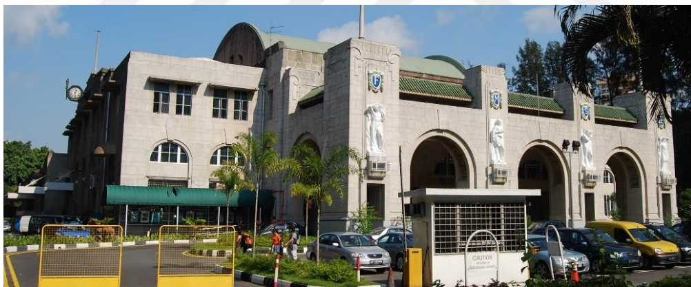
Figure 4.29 View of the vaulted roof on Tanjong Pagar Station [93]
