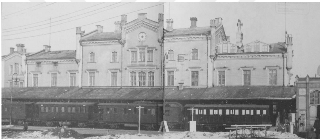
Figure 2.34 The rear façade of the Helsinki Old Railway Station [53]
