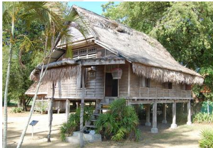
Figure 4.119 The Malay house of timber construction and gabled roof [168]
