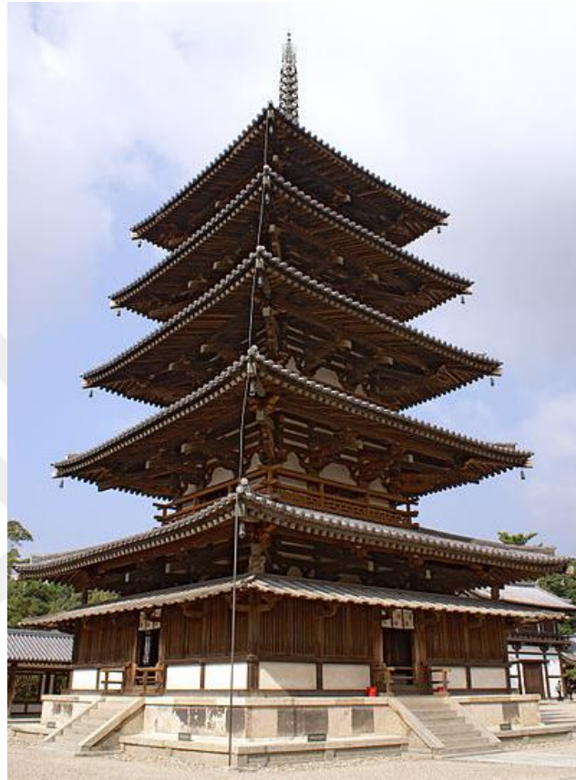
Figure 4.67 Decorative finial were place on top of the roof [147]
