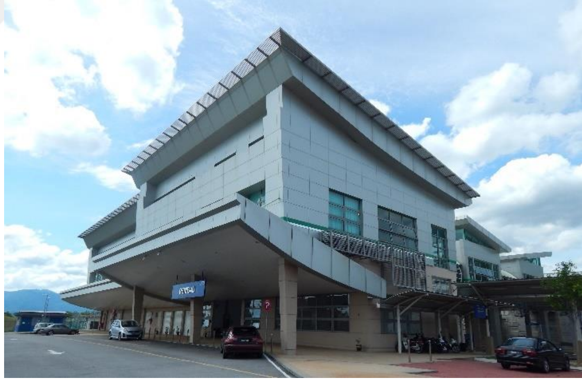
Image 114 The newly operated Rembau Station
