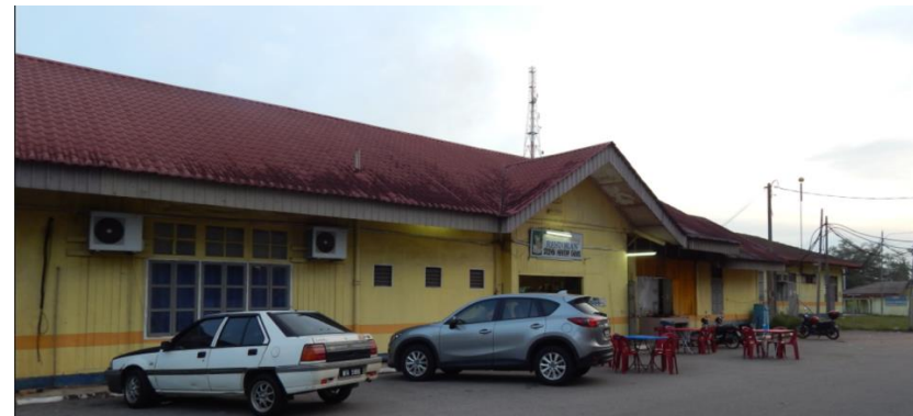
4. The right hand sides of the building are still occupied with the old restaurant
