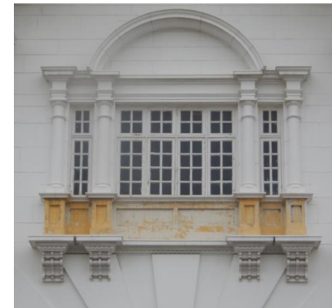
4. Tripartite Palladian windows; six panels of casement windows with Palladian style circular pediment trim and window sill together with support brackets
