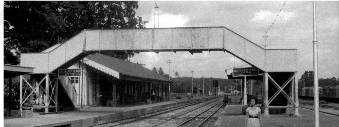
Image 116 Tampin Station looking north with overhead pedestrian bridges [71]
