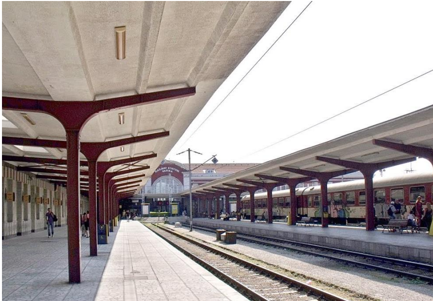
Figure 2.43 The combinations of concrete and steel columns were used for butterfly train-shed [59]
