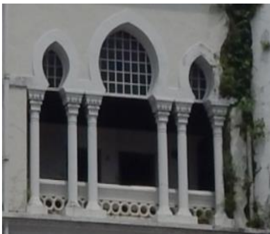
Figure 4.86 The pointed tripartite horseshoe arches in Kuala Lumpur station building
