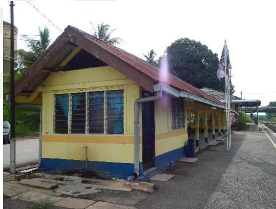
Image 131 View towards the ticket office
