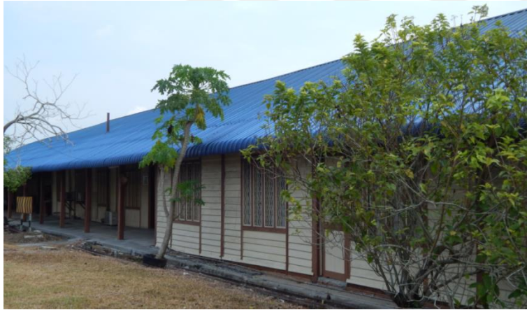
1. The old station was preserved but the roof has changed from its original.
