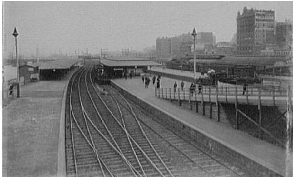
Figure 2.24 Australia Flinders Street Station 1895, Melbourne station [45]
