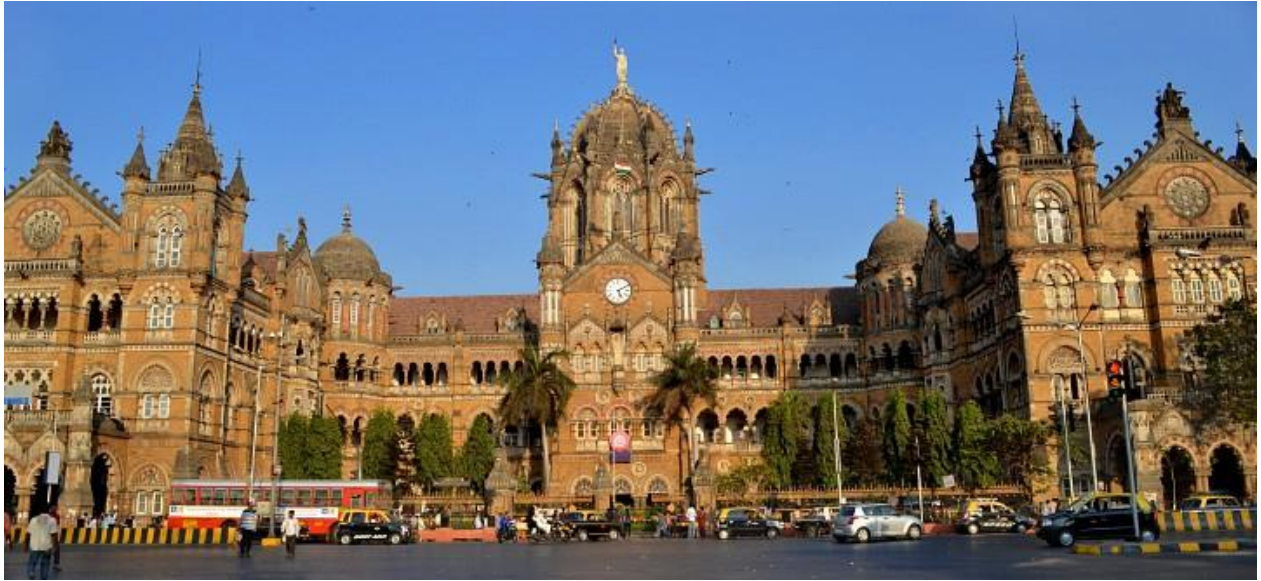
Figure 2.16 Façade of Chhatrapati Shivaji Terminus [39]
