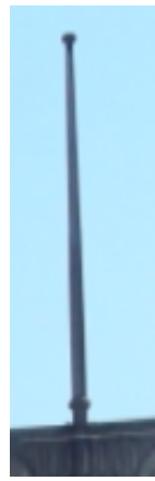
Figure 4.74 Flagpole finial at Tanjong Pagar station
