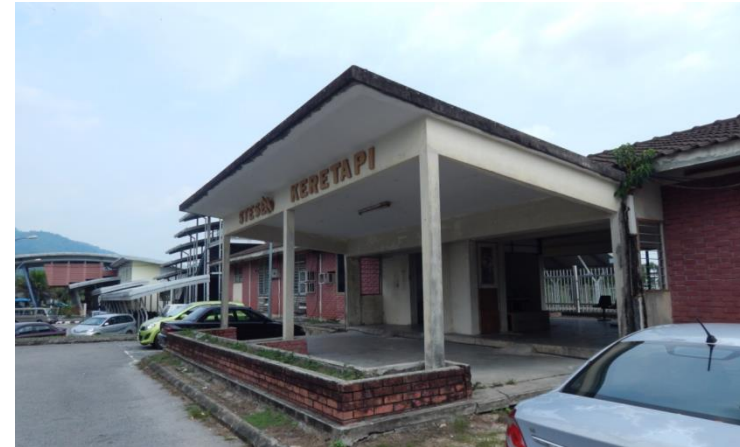
2. The portico of one storey station building.
