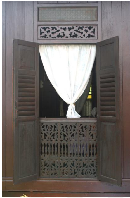
Figure 4.103 Traditional Malay house having long window panel with upper part having decorative elements creates better and natural ventilations [161]
