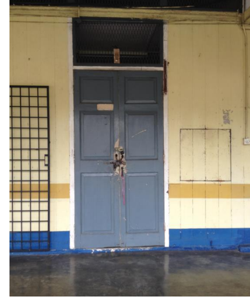
3. The image of two panels' timber door with wire-mesh at the upper door for ventilations
