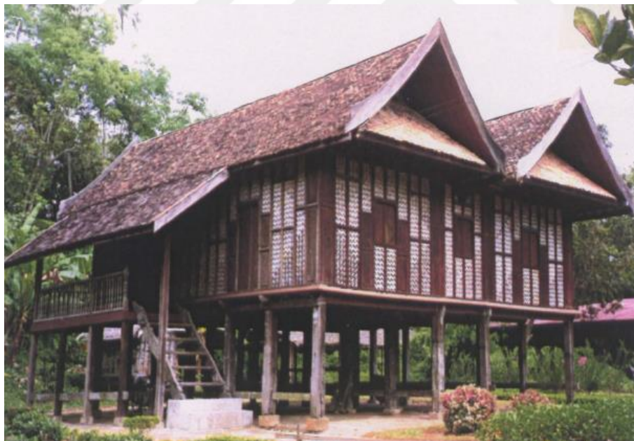
Figure 4.19 Typical gabled roof or ‘bumbung panjang’ in a Malay house [30]
