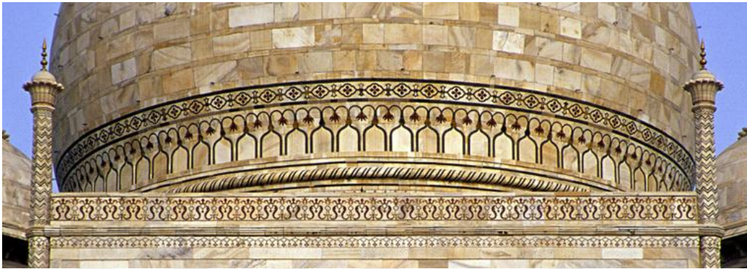
Figure 4.66 Guldasta, the ornamental pinnacle located at both ends of the cornice on top of the entranceway, [145]
