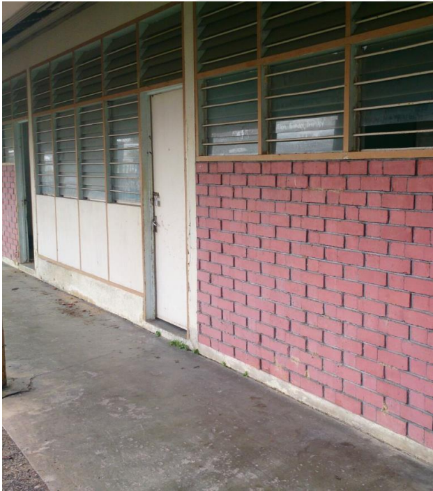
1. Single timber panel door and louvered glass panels windows.
