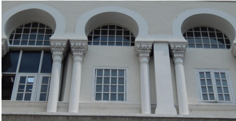
1. Horseshoe arches with double columns of Muqarnas capital were used at the station building.
