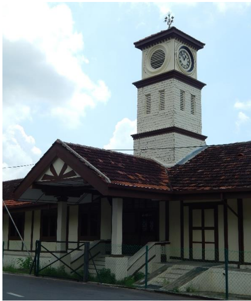
Figure 4.61 The Alor Star Stations' clock tower having square planned and pyramidal roof topped with finial
