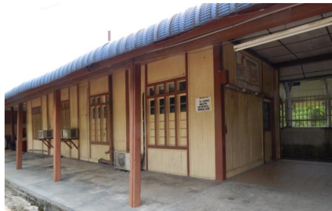
5. The view towards the office area.
