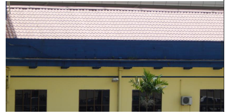
6. Parapet roofs in blue surrounding the building
