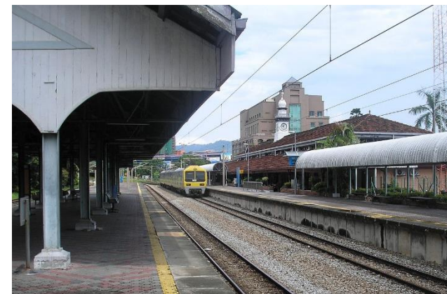
4. The steel columns and timber panel coverings as trains-shed
