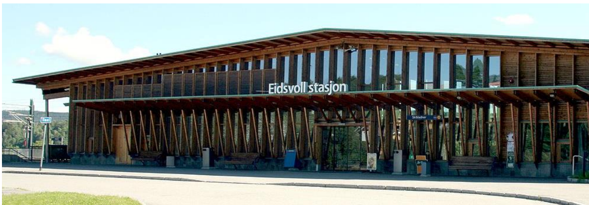
Figure 2.23 Façade of New Eidsvoll Station, Norway [44]
