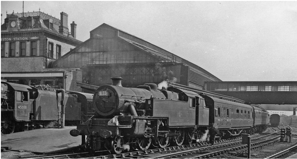
Figure 4.10 Preston Railway Station train-sheds' resembled the old Kuala Lumpur station train-sheds [114]
