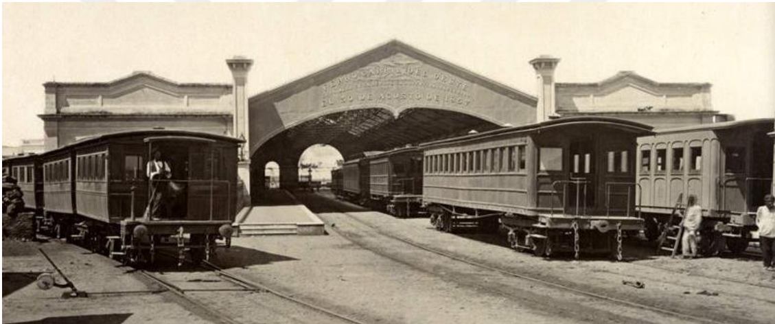
Figure 2.28 View of the train-shed from the west elevation of Del Parque Station [47]
