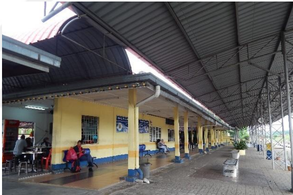
Image 97 View towards the restaurant and platform
