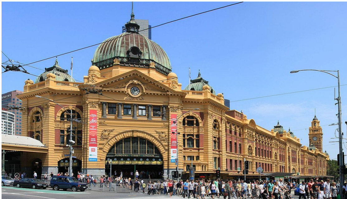
Figure 2.25 Current view of Flinders Street Railway built in 1900-1907 [45]
