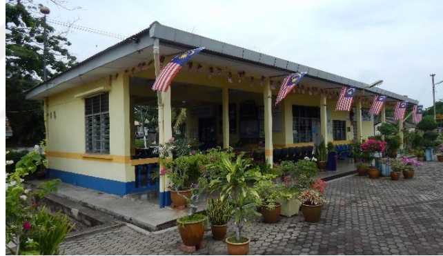
Image 135 View of the station from the track
