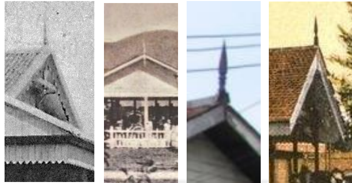
Figure 4.69 5 station buildings using the same pattern of rod type finial
