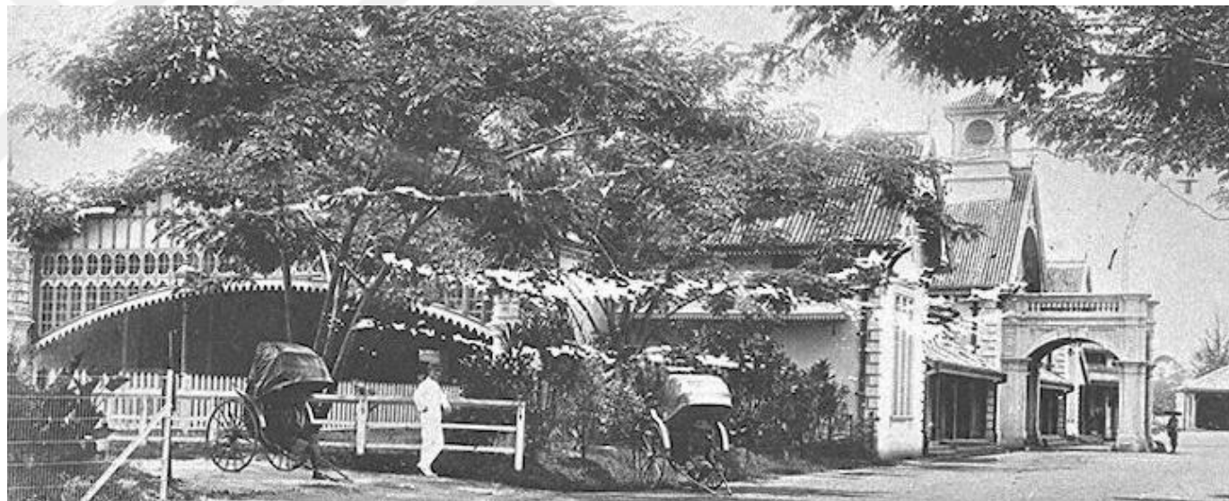
Image 11 View of the station building towards the loggia [71]
