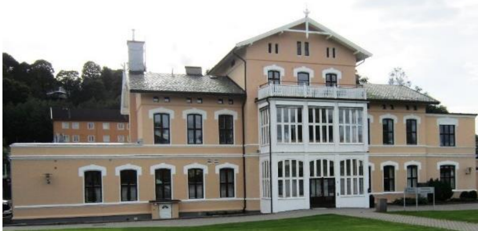
Figure 2.22 Façade of Old Eidsvoll Station, Norway [43]
