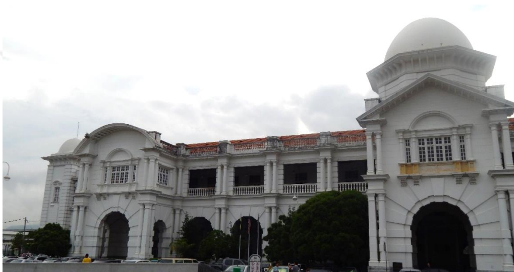
Figure 4.111 Balustrades along the roofline acts as parapet in Ipoh Railway Station
