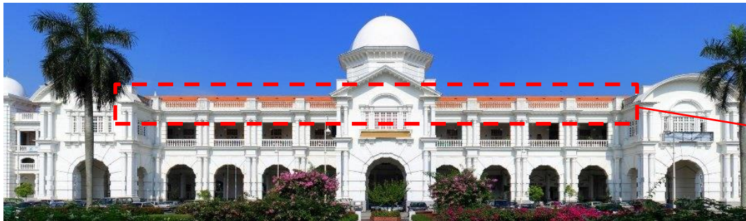
3. Overall view of the building façade showing balustrades on the roofline
