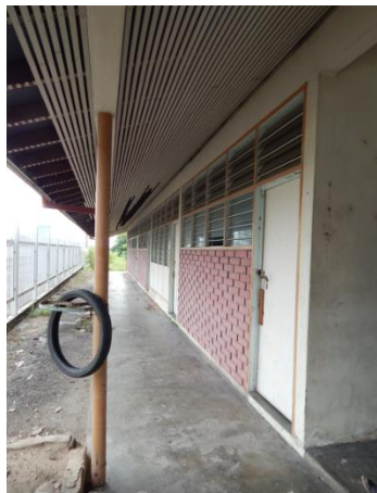
3. Louvered glass panel windows used on both; lower and upper part.
