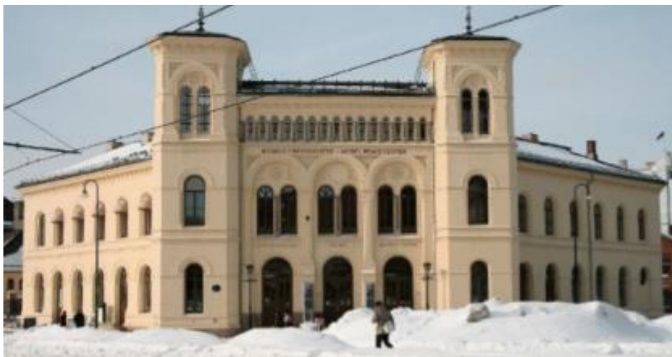
Figure 2.20 Image of Oslo West Railway Station [42]
