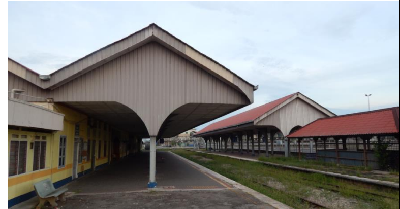
2. The image of the platforms and covered train-sheds which furnished with timber strips
