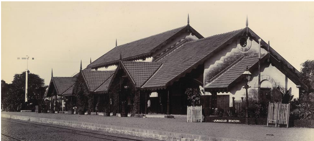
Figure 4.20 The 1895 view of Junagadh Station, India on application of gabled roofs [117]
