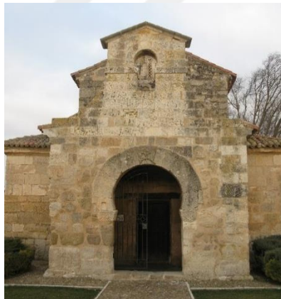
Figure 4.84 View of horseshoe arch on the west door of San Juan de Banor Church in Palencia, Spain built in 661AD [157]
