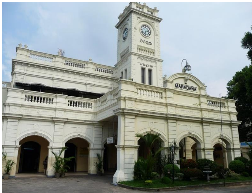
Figure 2.46 New station called Maradana Station, 1908 [61]
