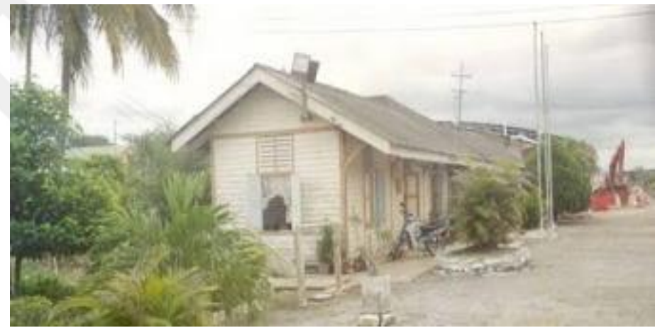
Image 108 View of the station.
