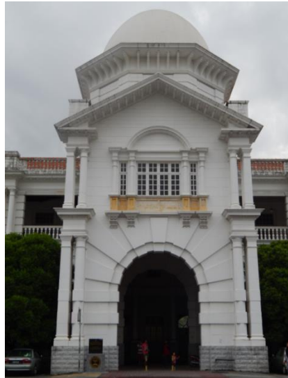
3. Projecting porch with Voussoir arch and tripartite Palladian windows on top of it
