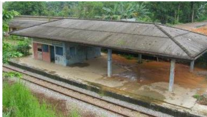
Image 150: View from the top of the station [76]
