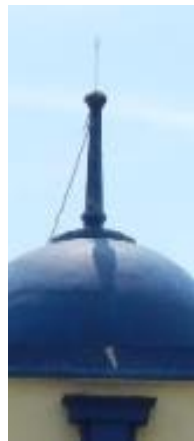
Figure 4.73 Flagpole as finial at Johor Bharu station
