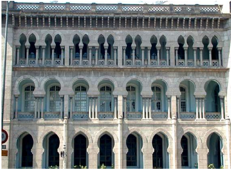
Figure 4.96 Pointed horseshoe arches on the ground floor, horseshoe arches of first floor and the twin series of pointed horseshoe arches on the second floor at KTMB Headquarters building, Kuala Lumpur Malaysia
