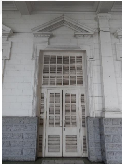
2. Double panels timber louvered doors with two fixed louvered panels on both sides. The upper part lattices are timber louvered.
