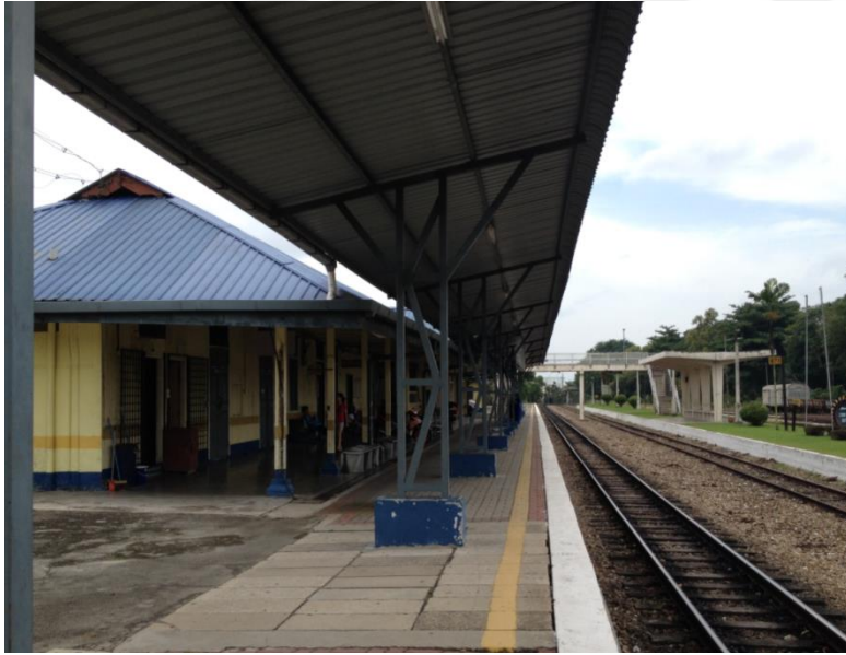
1. The image of the station with new roof being changed with blue metal decking and newly added butterfly train-sheds at the far right
