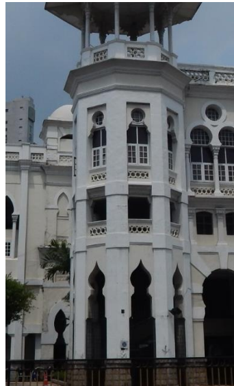
1. Ogee arches on the ground floor.
