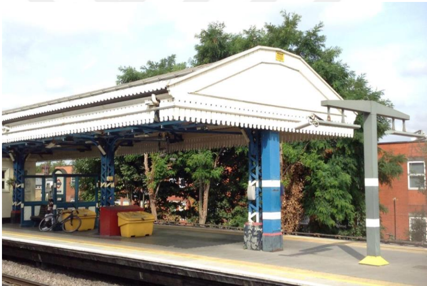
Figure 4.7 Turnham Green stations' train-sheds with steel column and timber panels as coverings
