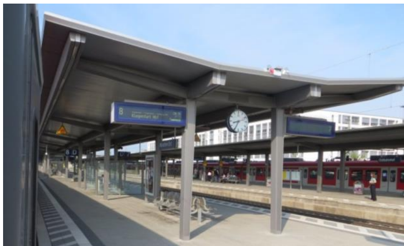
Figure 4.18 Munchen East Station, Germany shows the butterfly train-sheds
