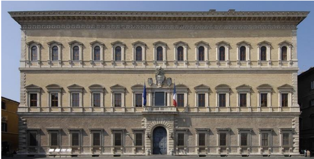
Figure 4.123 Triangular pediment windows broken at the lower part towards window panels, Palazzo Farnese, Rome [175]
