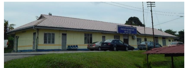
Image 145: View towards the station from the main road
