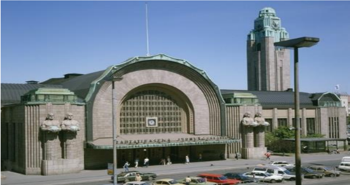
Figure 2.38 Current Helsinki Central Railway Station [54]
