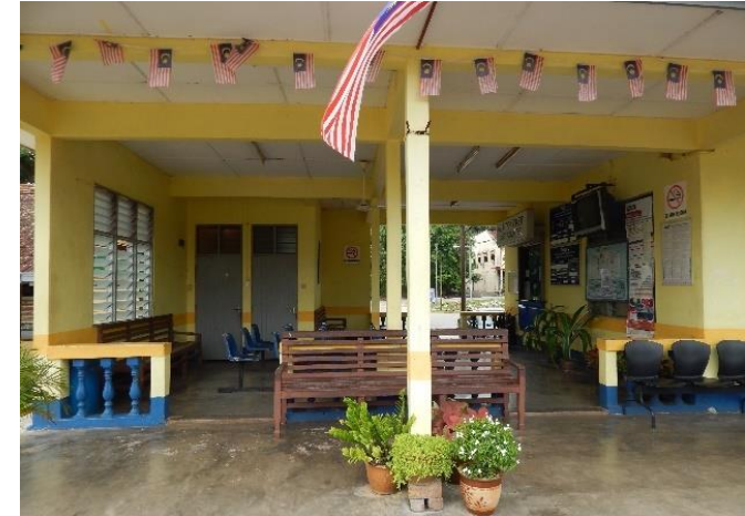
Image 138 View of the waiting area, ticketing office and toilets
