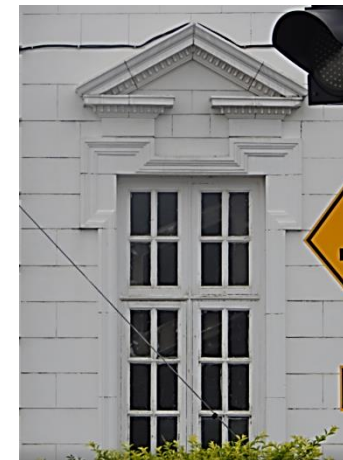
5. Double panels casement windows with triangular pediment as its trim
