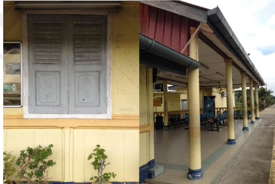
3. The two panelled timber windows with louvered on the top half,
