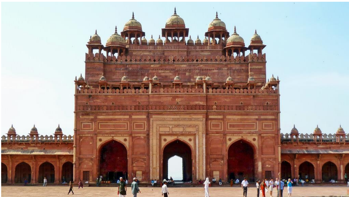
Figure 4.121 The portico with lavished ornamentations such as chatris, battlements, mini onion-shaped domes and guldasta of the Buland Darwaza's great gate in Agra, India [171]
