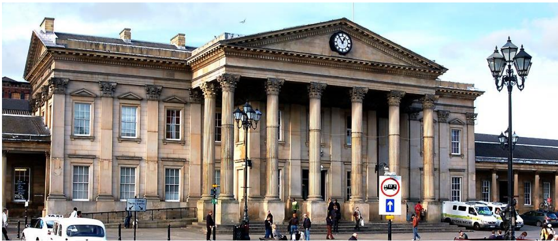
Figure 4.105 Huddersfield Station, England seen with porticos and windows of triangular pediment trims, [163]
