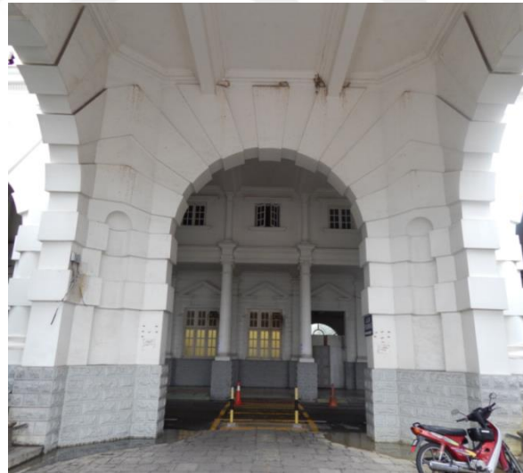
2. Overlooking through the porch.
