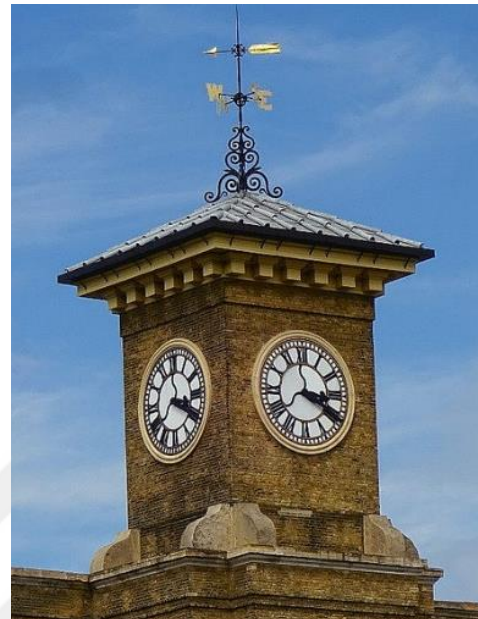
Figure 4.62 The King's Cross Stations' clock tower with square shape and pyramidal roof topped with finial [144]
