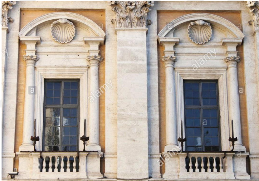
Figure 4.124 Segmental pediment windows broken at the lower part towards window panels, Campidoglio Palace, Rome [176]
