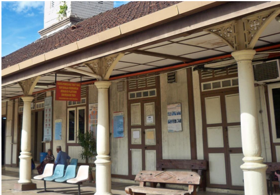
Figure 4.56 The concrete columns with decorative steel knee braces of floral motifs [139]
