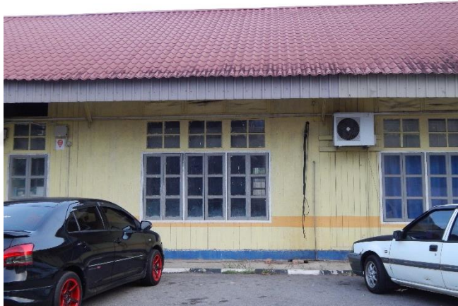
1. The timber panel window has been changed to timber glass panels windows
