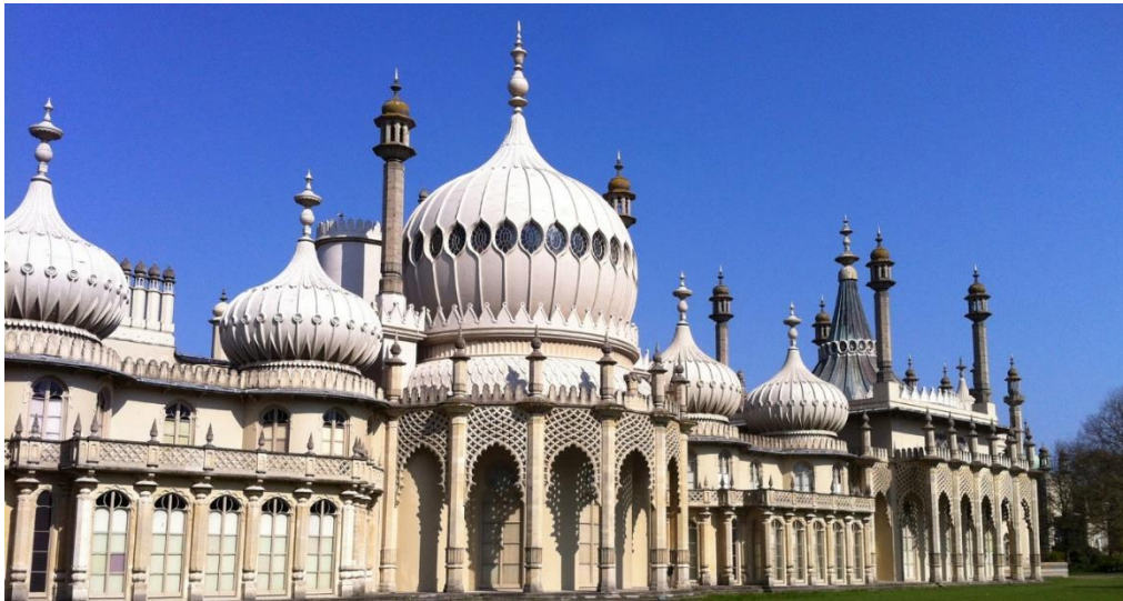
Figure 4.44 Royal Pavilion in Brighton Great Britain applied onion domes in various sizes [134]
