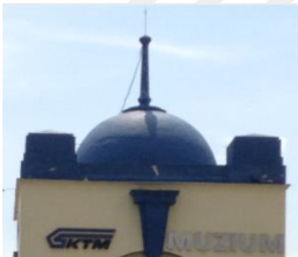
Figure 4.34 Hemispherical dome on Johor Bharu station
