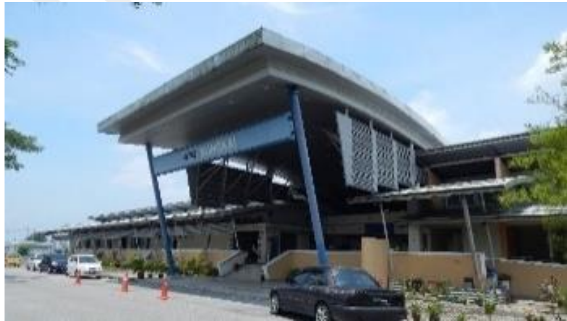
Image 107 View of the new station
