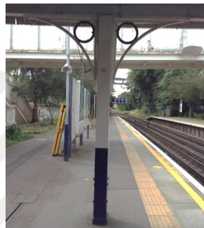
Figure 4.50 Kew Garden Station in London had the same column and knee braces like in Taiping Station, Perak
