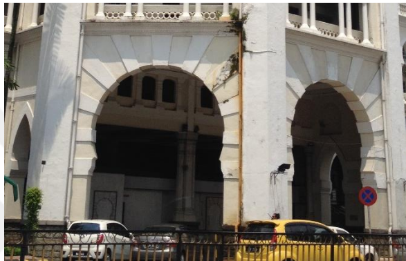
Figure 4.98 Voussoir horseshoe arches in Kuala Lumpur station building applied similar approaches on its wall appearance
