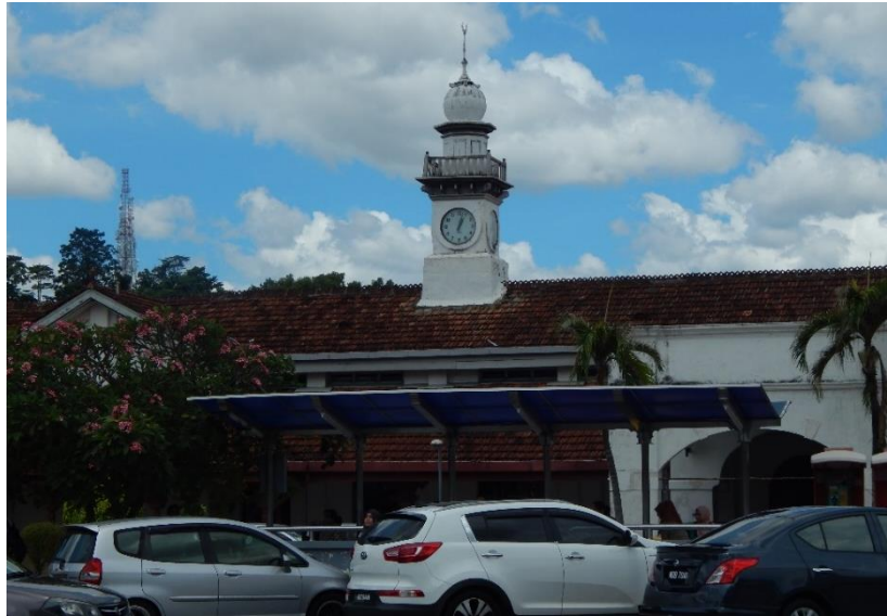
Figure 4.59 The clock tower with square planned with balustrades all around as parapet and topped with onion dome at Seremban station
