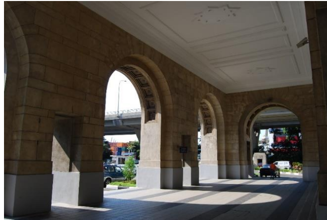
Figure 4.100 The interior view of the voussoir arches at Tanjong Pagar Station [129]
