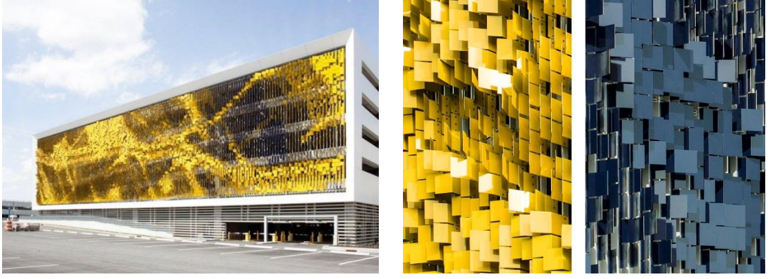
Şekil 3.8 Eskenazi Hospital Parking Structure cephesi [62]
