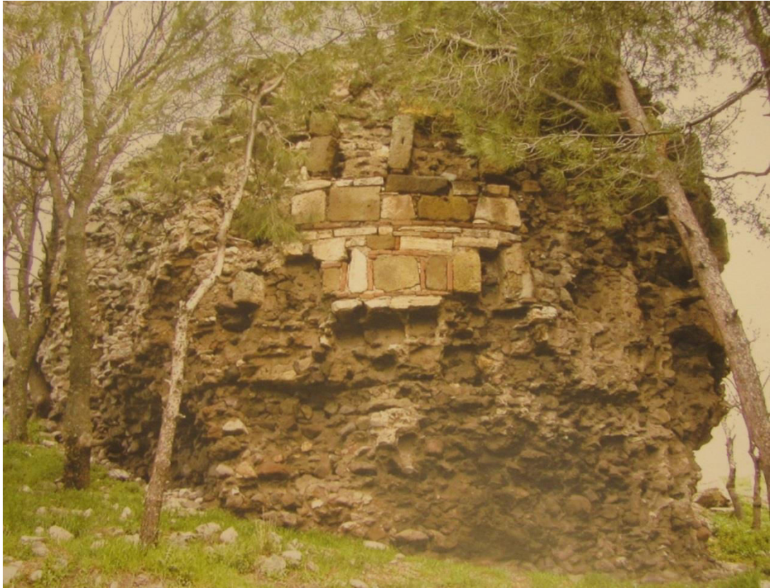
Figure 40: Pegadia wall detail (Mercangöz, 2003: 39)
