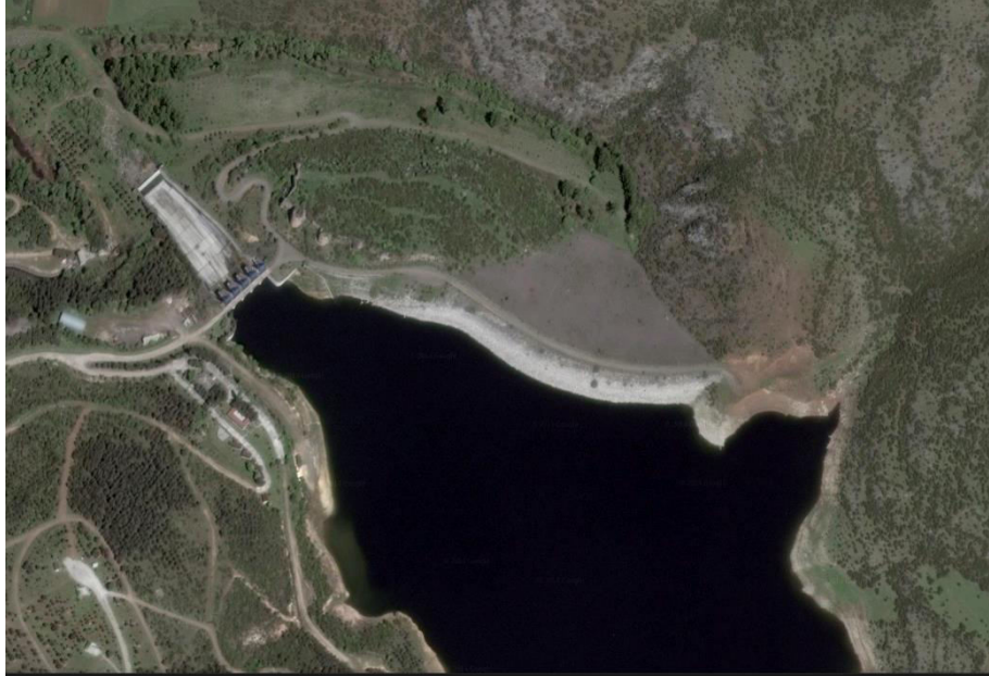
Figure 37: Satellite view of Achyraous-Esseron and the İkizcetepeler Dam (Google Earth)
