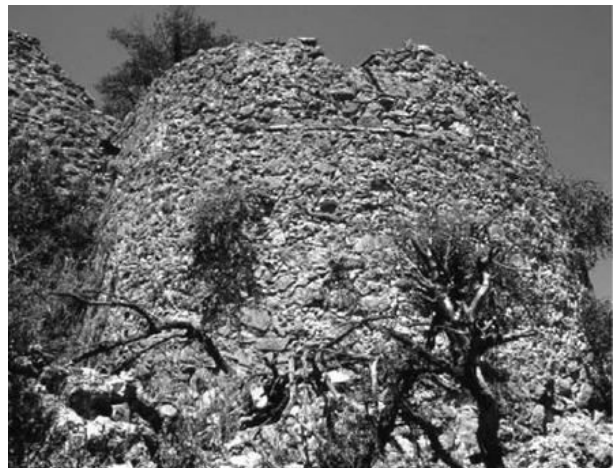
Figure 42: Tower at Yarbaşıandır (Akyürek, 2006: 16)
