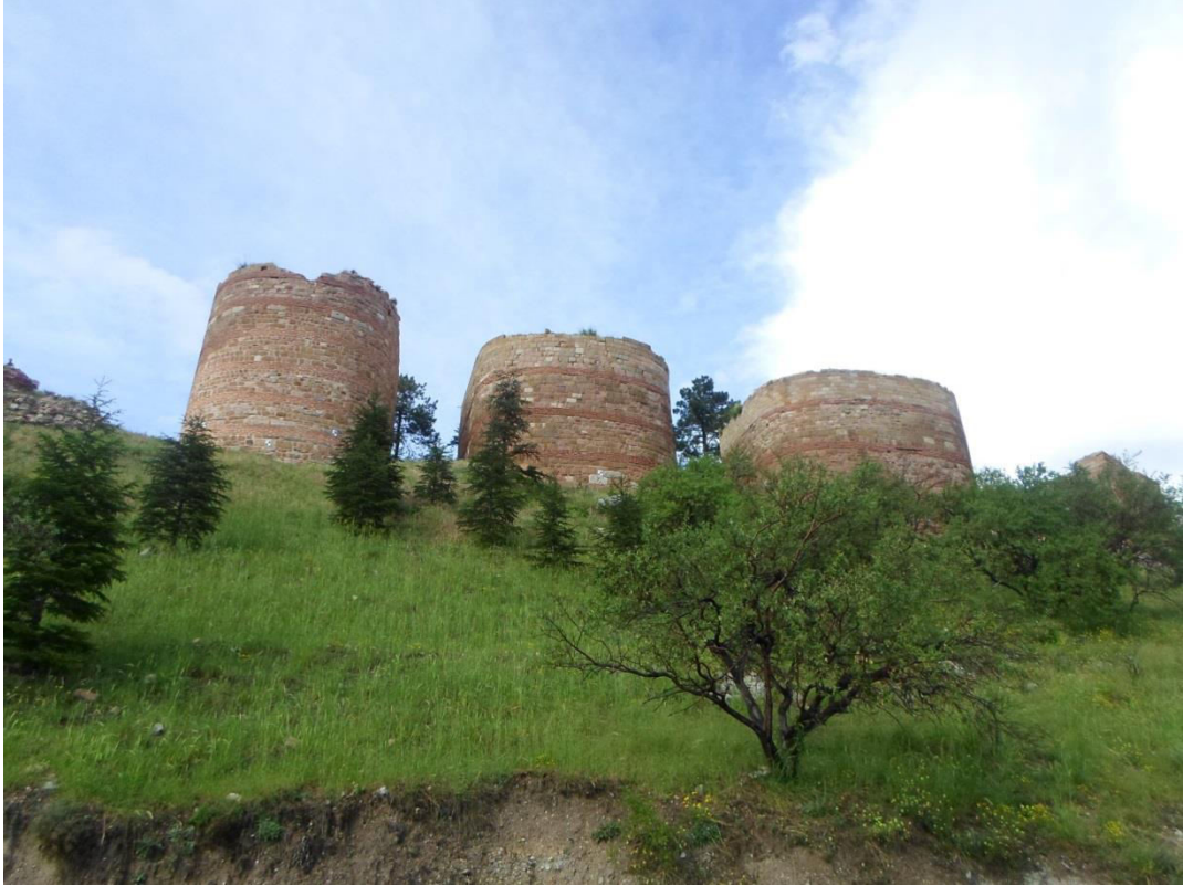
Figure 67: Closely spaced towers of Kotyaeion (Photo: N. Aktaş)
