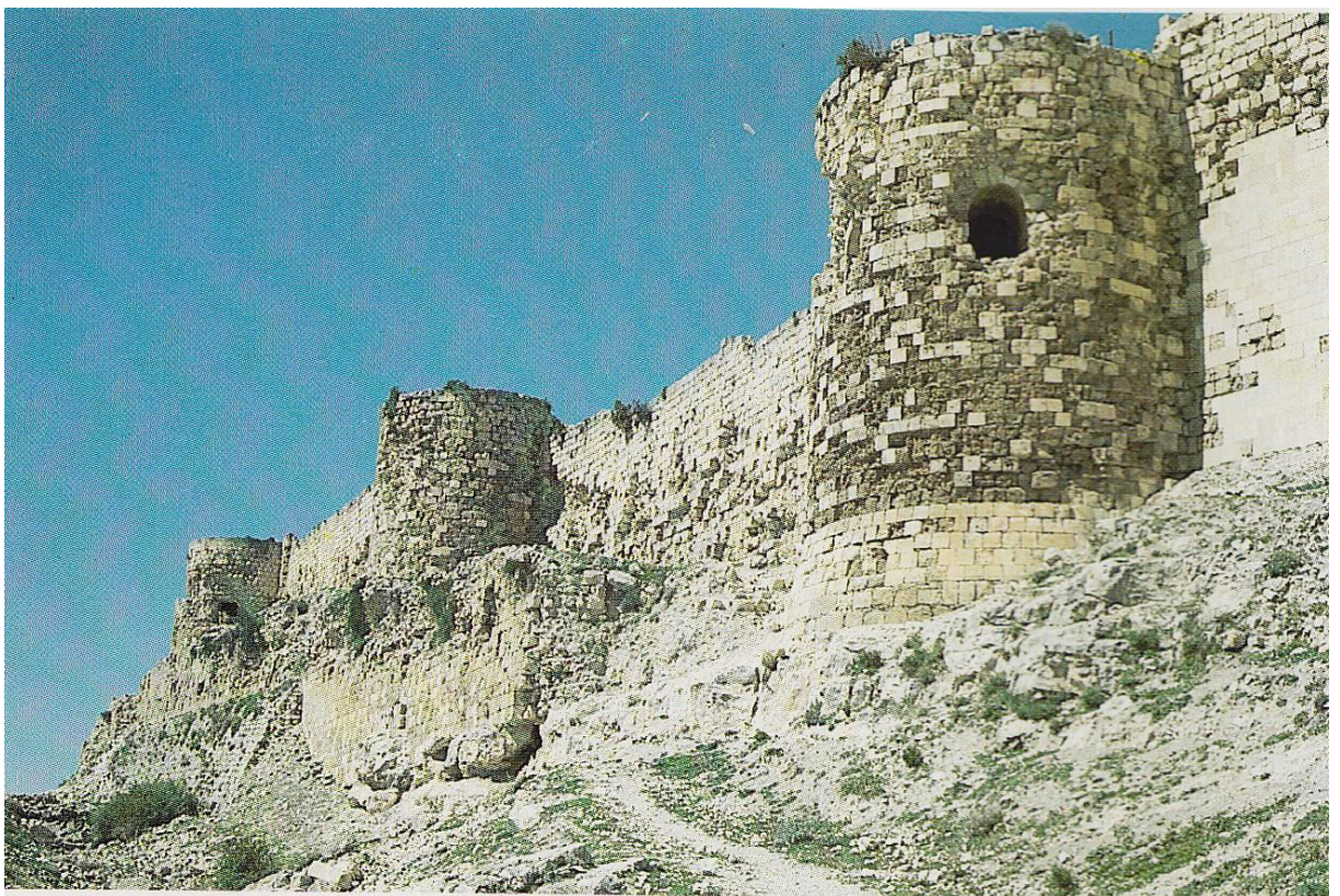
Figure 15: Walls of Seleukeia (Edwards, 1987a)
