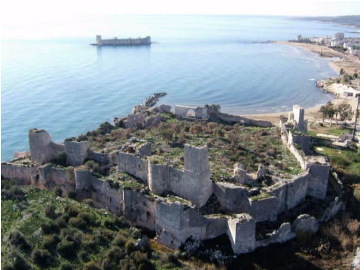
Figure 12: Korykos aerial view (Photo: B. Elliott)
