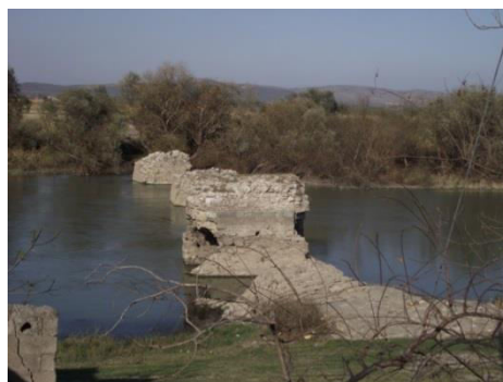
Figure 35: Makestos Bridge (Photo: Author)
