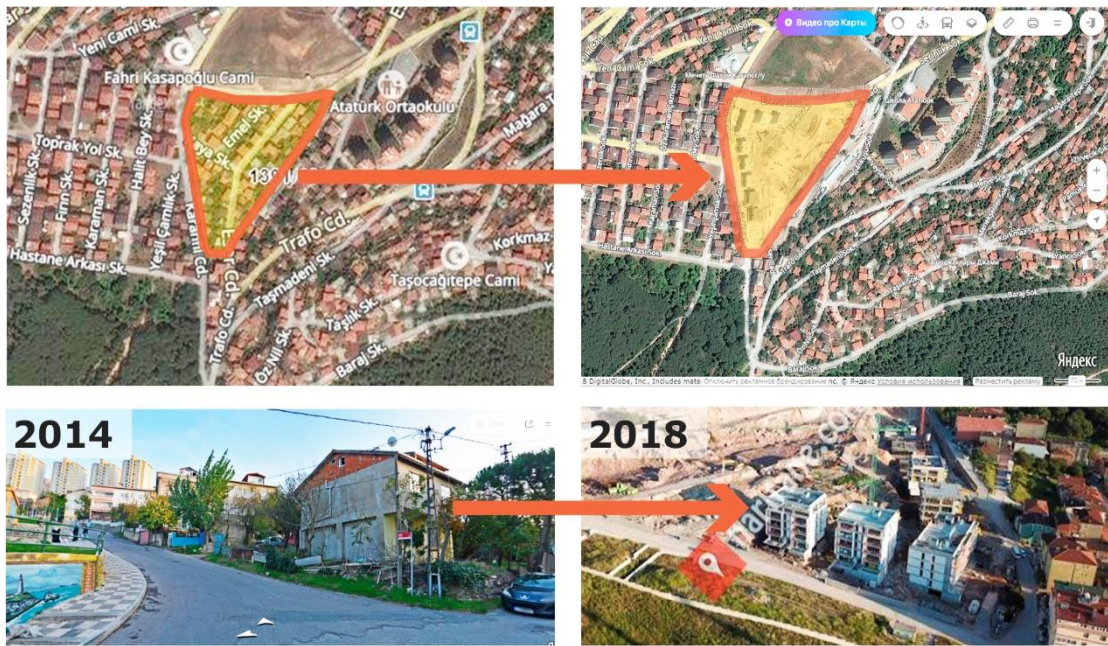
Figure 3.12 Basibuyuk Before and After the 2'nd stage Renovation
