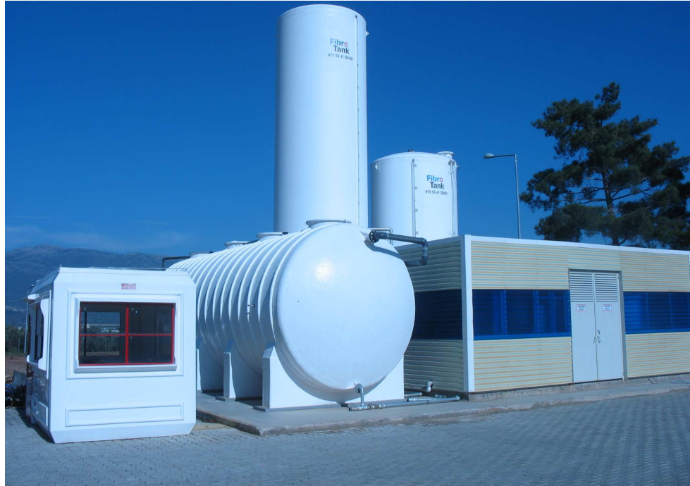
Figure 1.1 Industrial products made by GRP ( photo courtesy of Erdem Yucel, Fibrosan Inc., Izmir, Turkiye)
