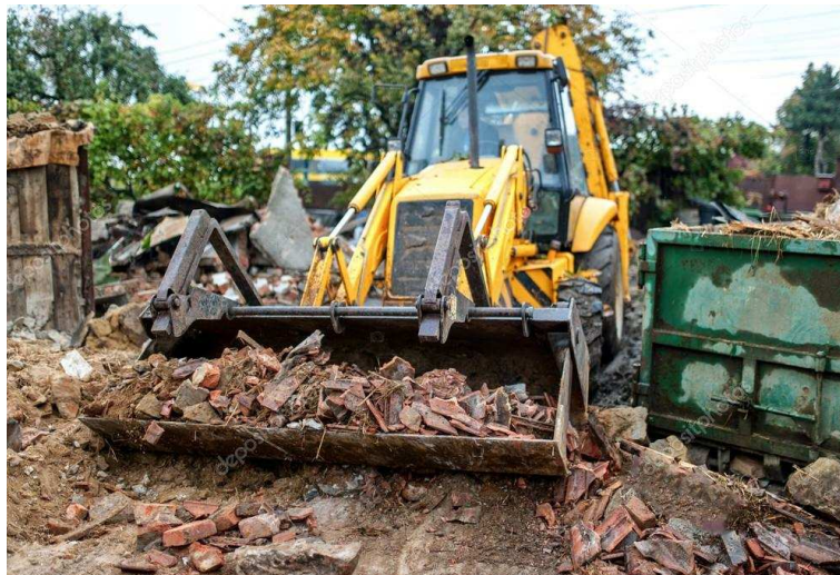
Figure 1.2 Dozer for Debris Removal
