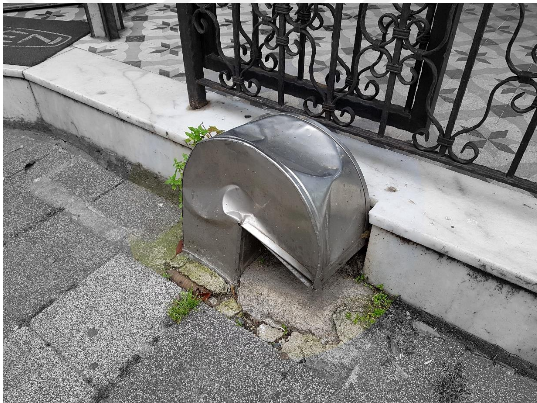
Figure 3.20. Traces of waiting on a ventilation duct (April 18, 2019)
