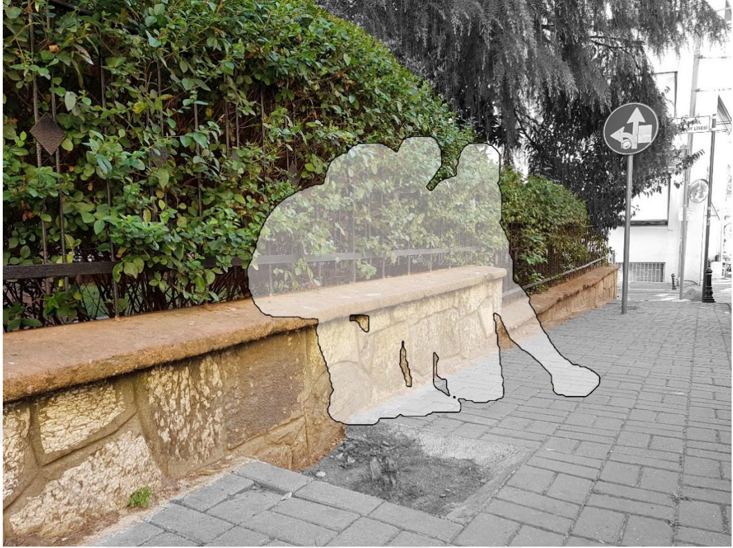
Figure 3.31. Informal placemaking on a wall (July 1, 2019)
