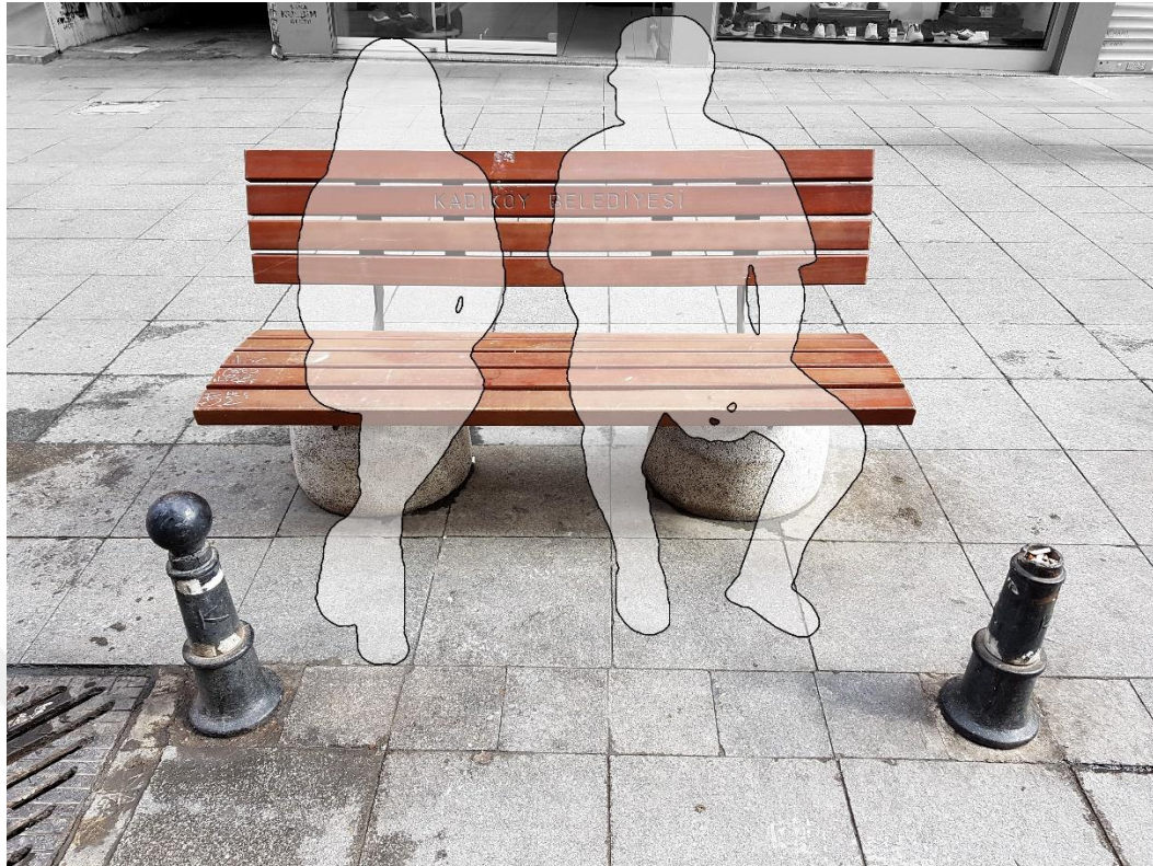
Figure 3.22. Bench with a broken pavement bollard (April 12, 2019)
