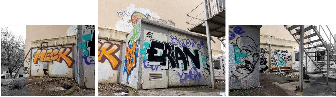
Figure 3.48. Graffiti area behind the former Kadıköy Şifa Hospital (April 12, 2019)
