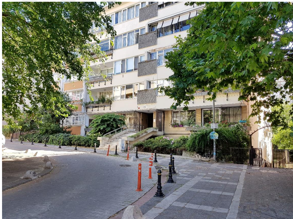
Figure 3.8. A view from residential area in Caferağa (July 1, 2019)
