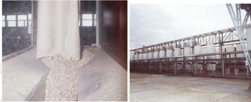
Figure 2-2. Extraction unit (TGB, 2013)
