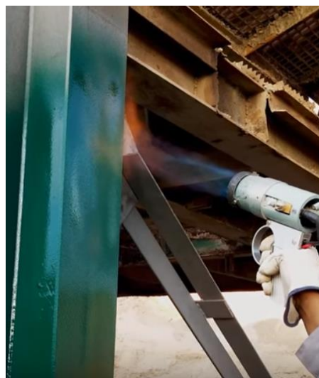
Figure 6 Flame spray application of powder paint on metal objects
