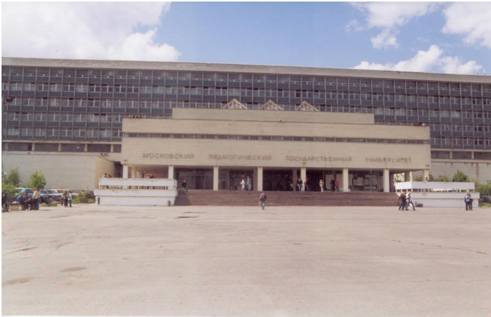
PHOTOGRAPH 1: (May, 2005) Moscow State Pedagogical University (MSPU) building and its courtyard, the main entrance, during the spring
