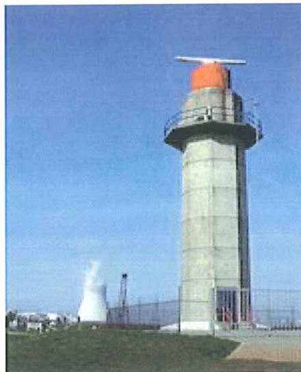
Figure 4.9 European Union vessel traffic monitoring
