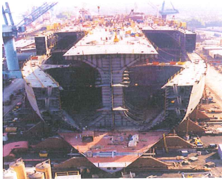
Figure 4.17 Building of double-hull tanker
