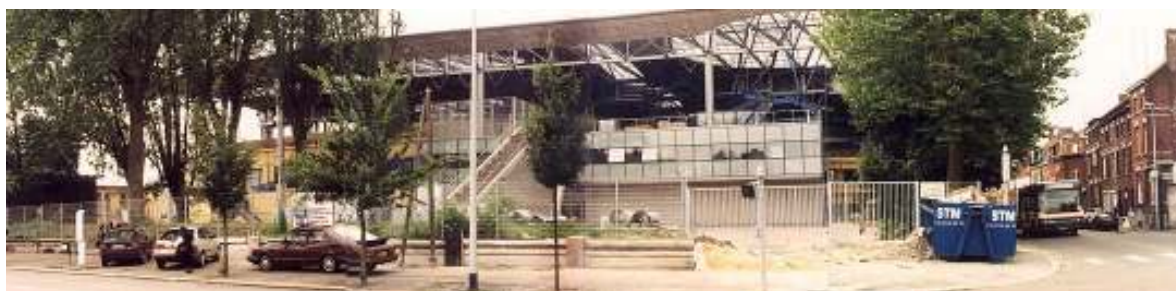
Figure 6.10. The façade of the National Studio for contemporary arts
