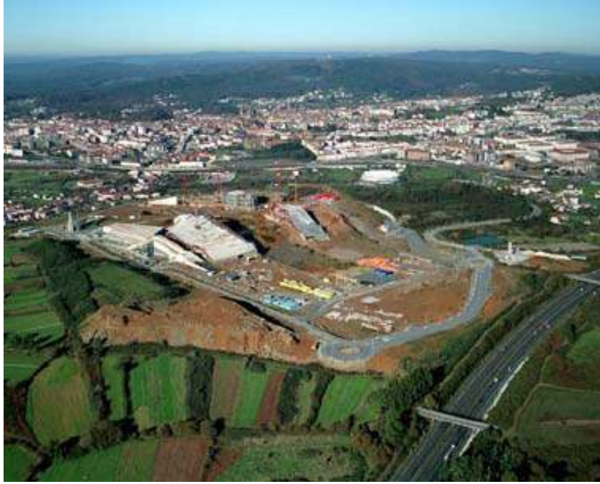
Figure 6.35. The above view of the construction area of Galicia
