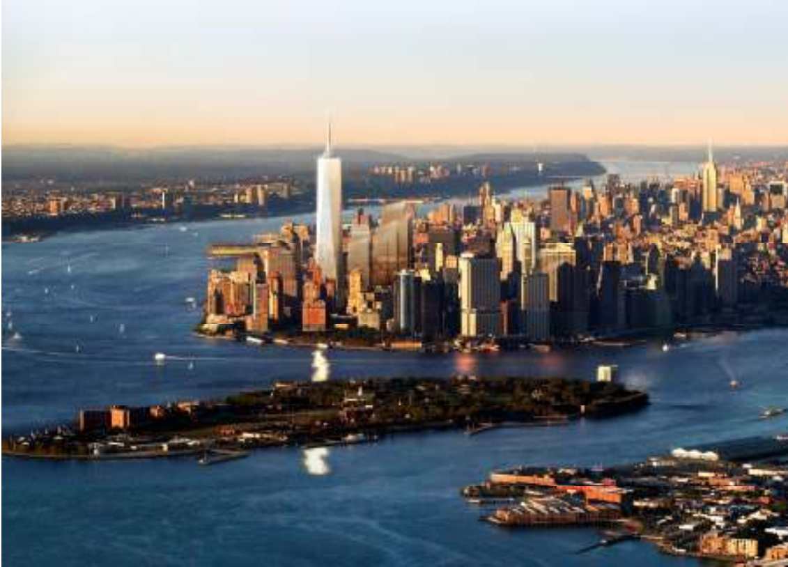
Figure 6.59. The silhouette of New World Trade Center http://www.renewnyc.com/images_WMS/freedom_tower/Harbour
