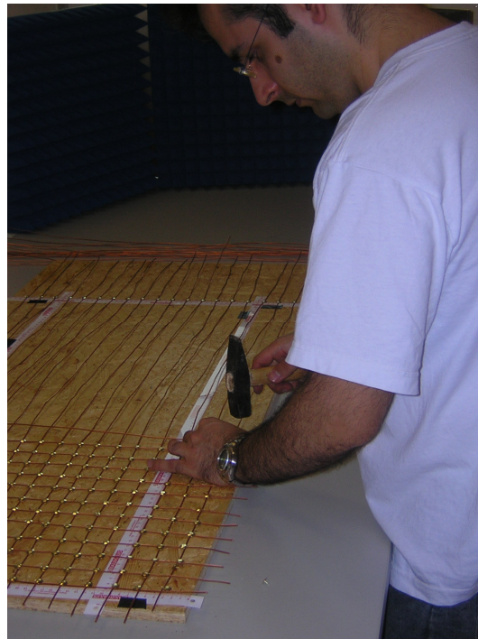
Fig.3.2.3.3.c: Rebar grid installation for flooring and ceiling
