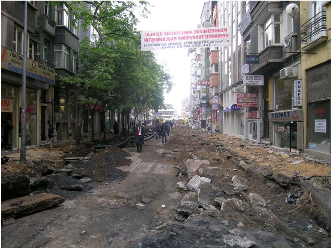
Picture 4.4 Paving Renovation Activities in Talimhane
