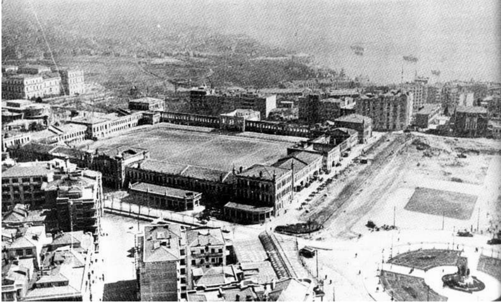
Picture 3.5 Taksim Barracks
