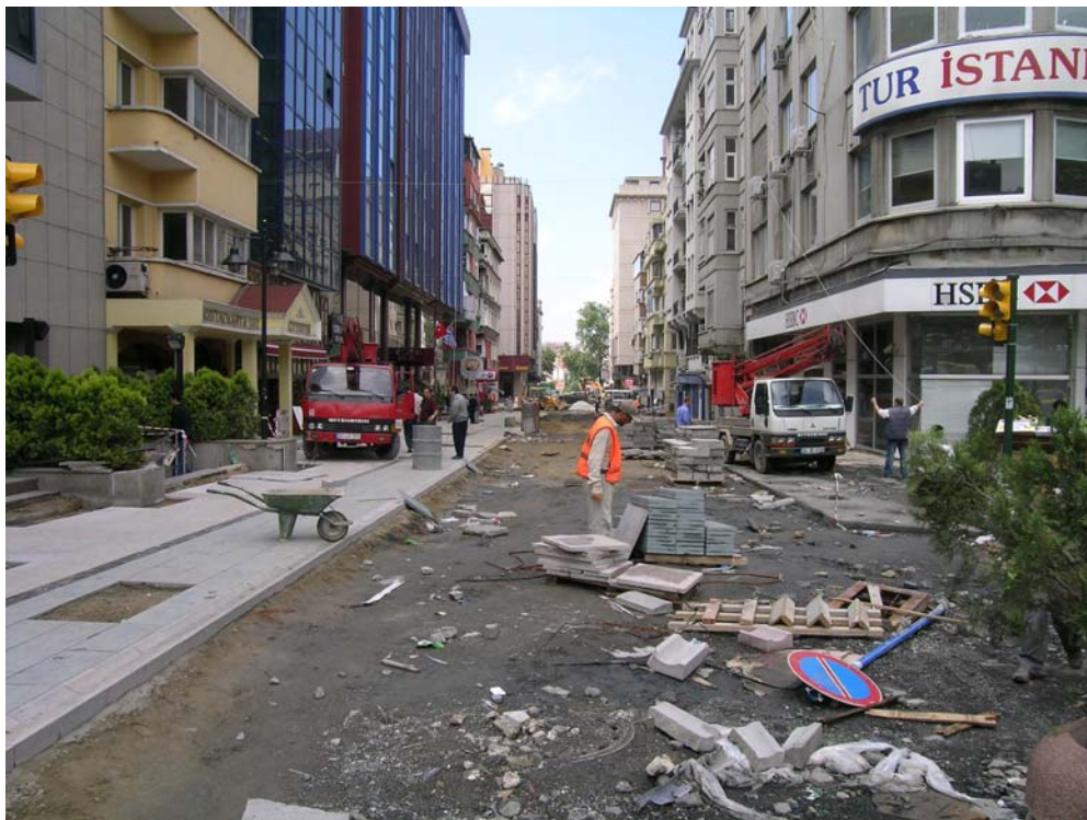
Picture 4.5 Renovation Activities in Talimhane
