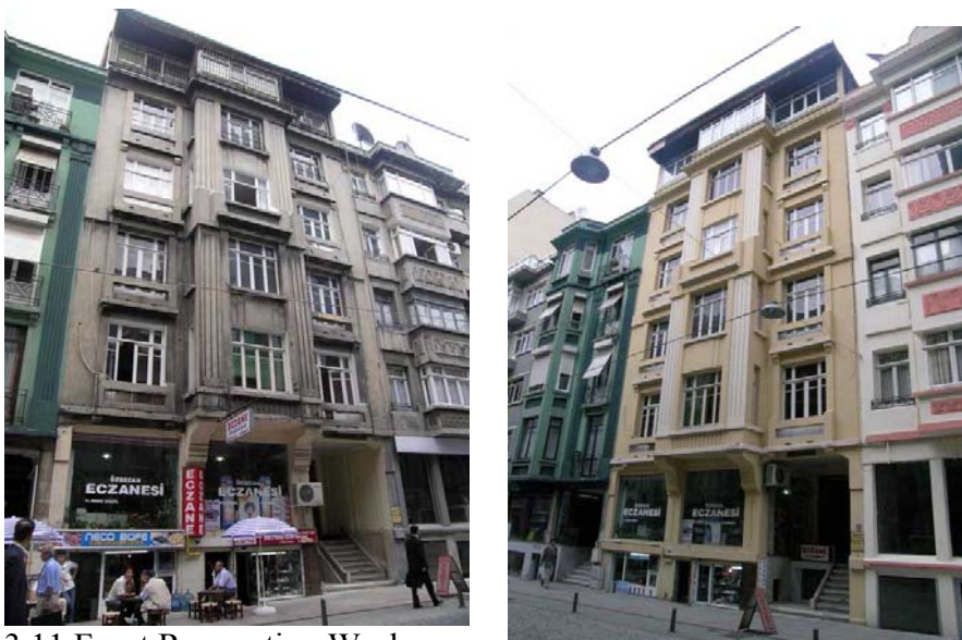
3.11 Front Renovation Works
