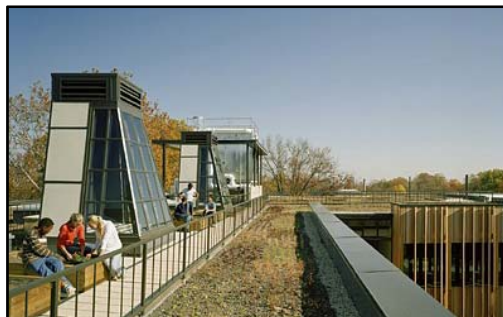
Figure 3.42. View of planted roof, garden, and solar chimneys [34]
