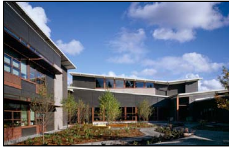
Figure 3.21. South courtyard with native plants and adjacent classroom cluster [47]
