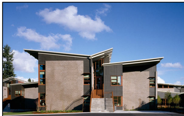
Figure 3.23. Classroom cluster from outdoor play area [47]
