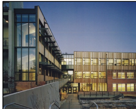
Figure 3.38. Reclaimed wood cladding was fabricated off-site in large sections [65]
