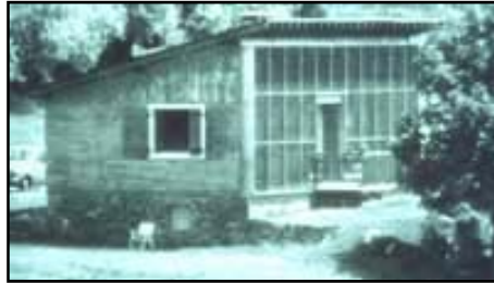
Figure 2.6. Original "Trombe" wall house in Odeillo, France, 1964 [19]
