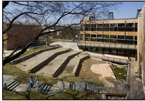
Figure 3.39. View from southwest overlooking wetlands courtyard [65]
