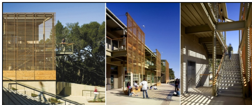
Figure 3.32. Sunshades on different facades [64]
