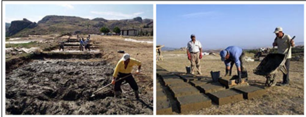
Figure 4.5. Preparing the adobe mixture and pouring it into the molds [35]
