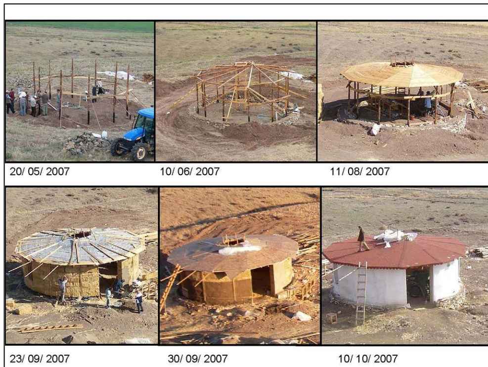
Figure 3.19. Construction stages of the meeting room
