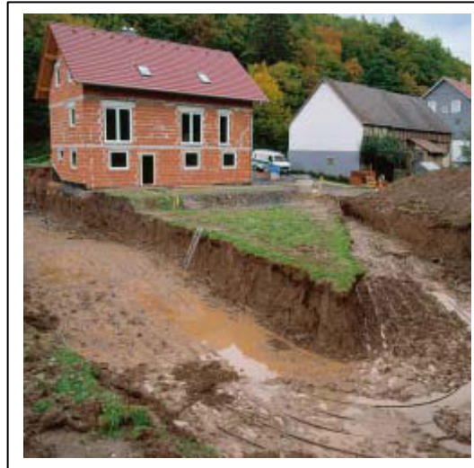
Figure 4.27. Producing heat with horizontal soil collectors [51]
