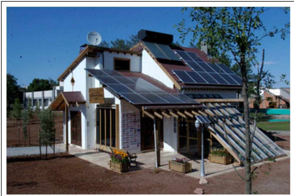
Figure 4.30. Diyarbakir solar house, a successful application; generates own energy [46]
