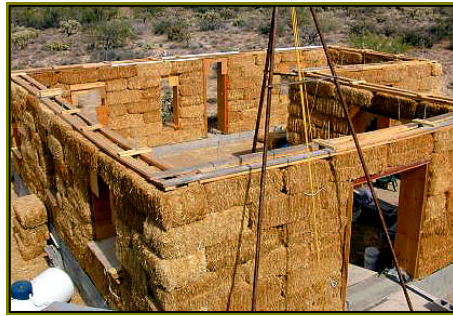
Figure 3.10.Straw Bale House Construction [50]
