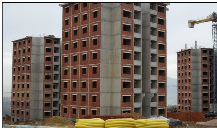
Figure 3.4. Typical Reinforced Concrete Construction for Residences [30]
