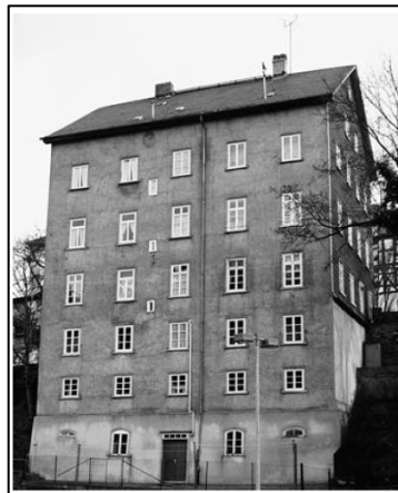
Figure 3.9. Rammed earth house, Weilburg, Germany, 1828[48]
