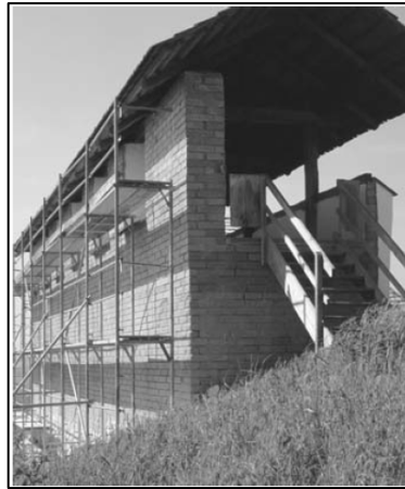
Figure 3.8. Reconstruction of mud-brick wall, Heuneburg, Germany, 6th century BC [48]
