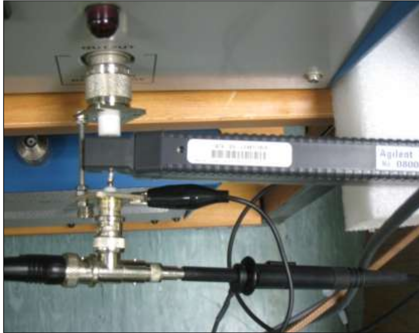
Figure 2.2. Connections on power amplifier output to current and voltage probes.
