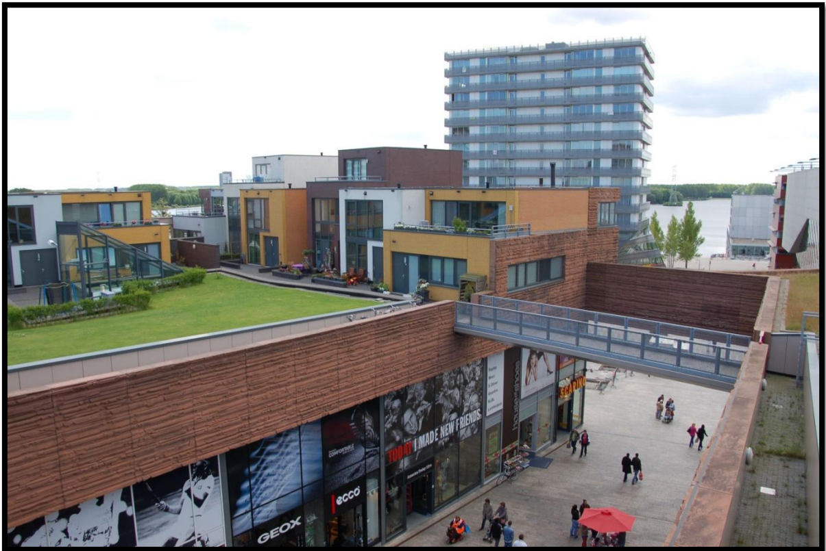
Figure 1: Use of the rooftop in the city of Almere [42]
