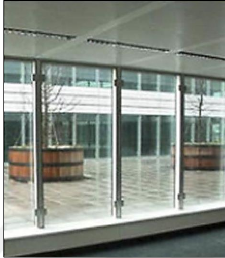
Figure 2.4. Corridor type double-skin façade [24]
