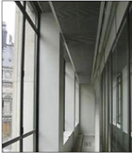
Figure 2.3. Shaft-box type double-skin façade [24]
