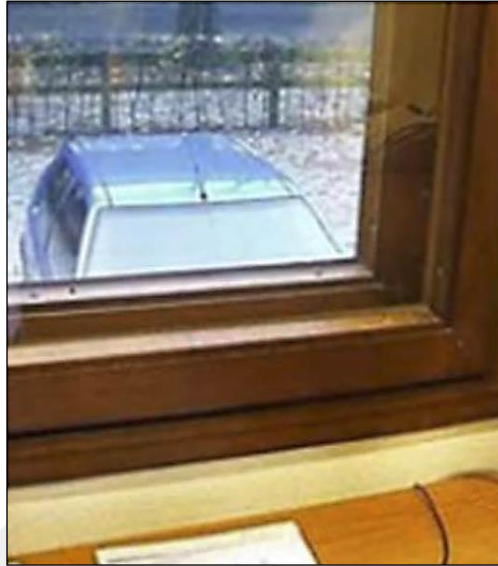
Figure 2.2. Box-window type double-skin façade [24]
