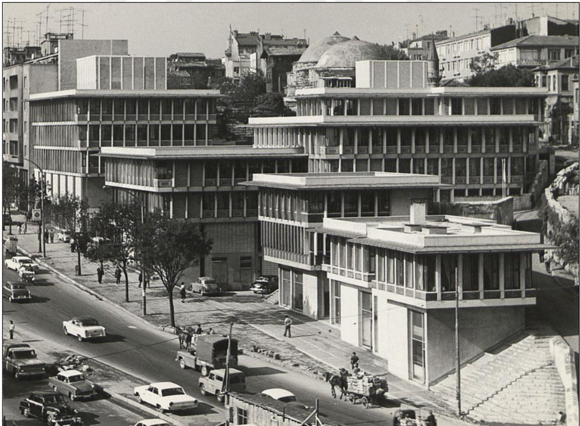
Figure 5.38. SGK Building, Rahmi M.Koç Archive, Salt Research
