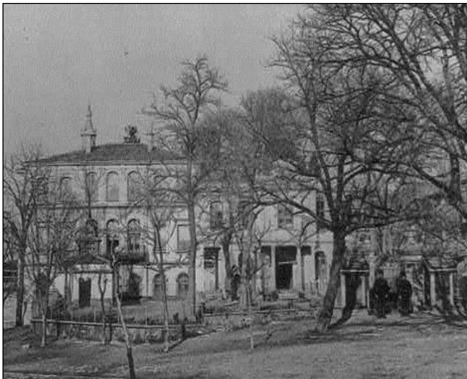
Figure 4.40. Imperial Police Station built at Vefa Meydan, 1880-1900, LoC
