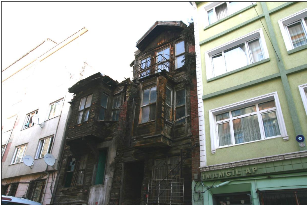
Figure 5.42. 19 th century housing units in Zeyrek, 2015, photo by the author
