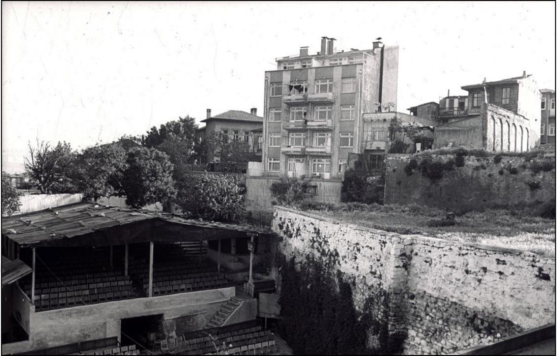
Figure 5.9. New apartment block in Zeyrek, circa 1970 , Kemali Söylemezoğlu Archive, Salt Research
