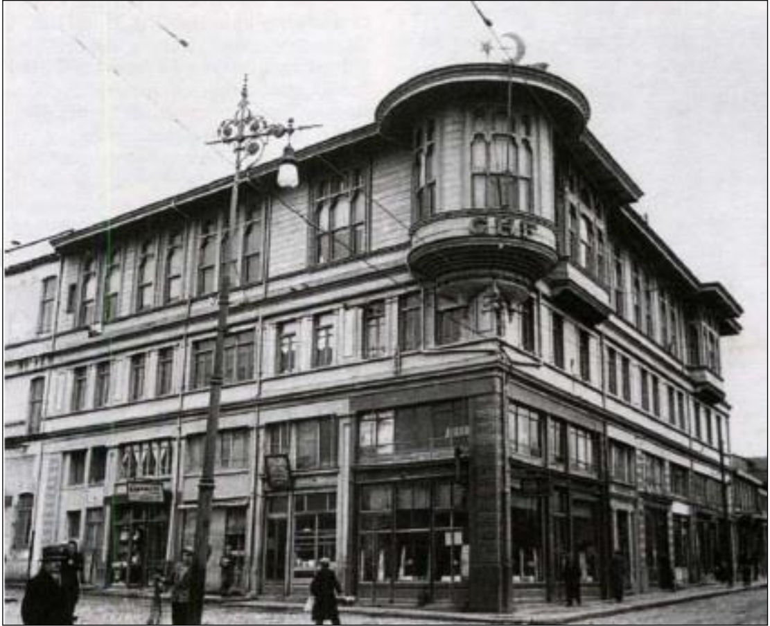
Figure 4.28. An apartment building in Şehzadebaşı [31]
