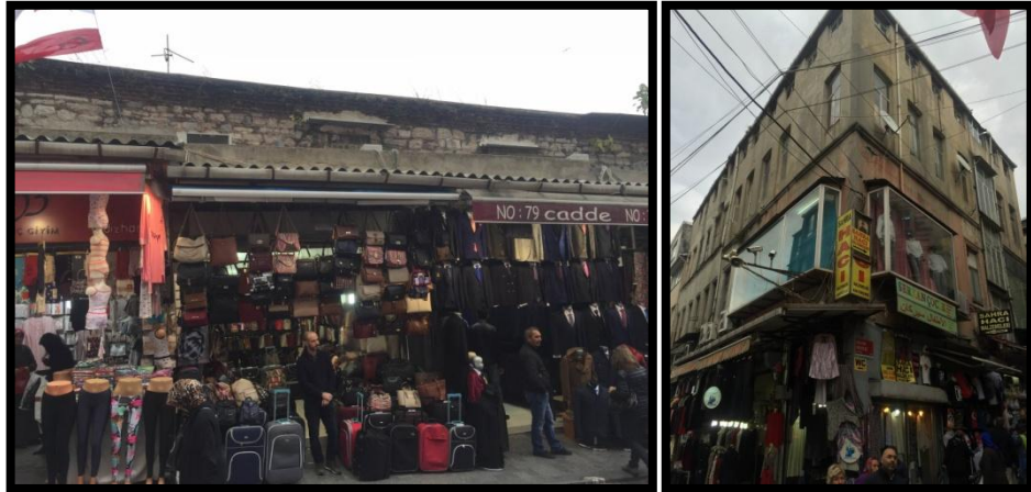
Figure 1.22. and Figure 1.23. Current view of Mahmutpaşa Street building additions [13]
