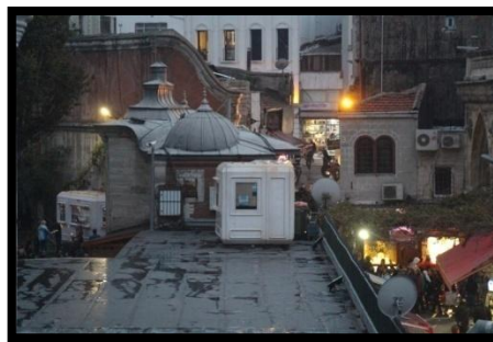
Figure 2.112. Booth view on the roof of back-courtyard of Nuruosmaniye Mosque [13]
