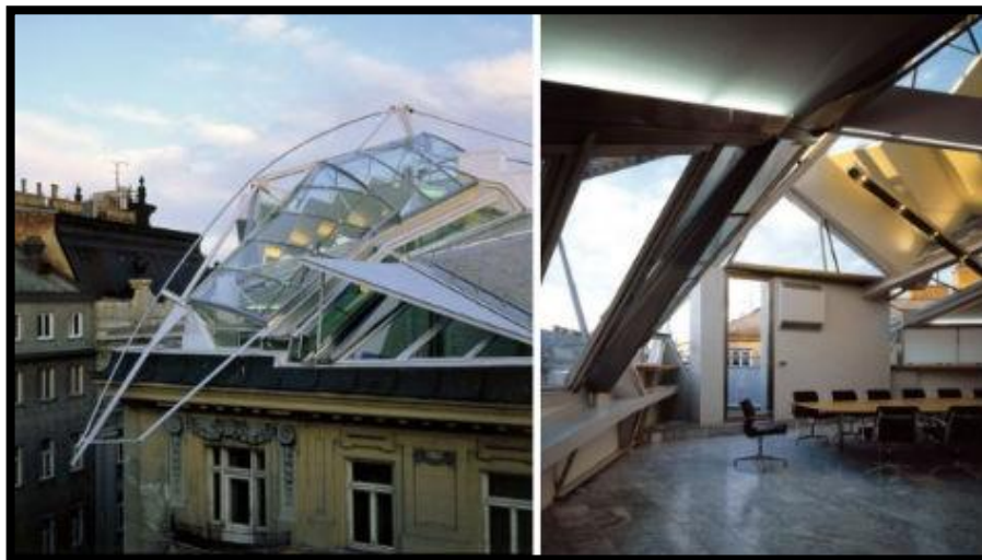
Figure 2.41. Rooftop Office in Vienne [56]
