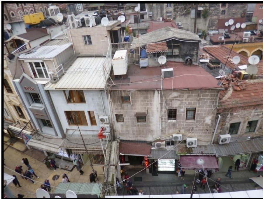
Figure 2.117. Rooftop add-on space view [13]
