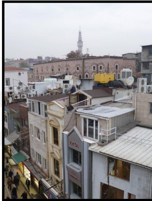
Figure 2.104. Ventilation and Chiller Tower on Rooftop [13]
