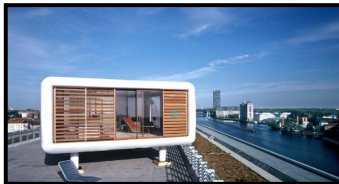
Figure 2.54. Loft Cube on a rooftop [68]
