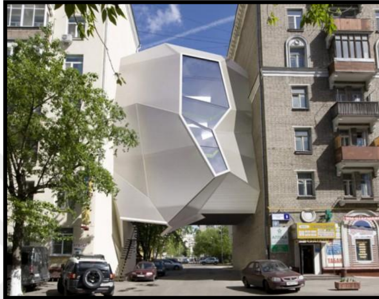
Figure 2.79. Hanging Parasite Office in Moskow [79]
