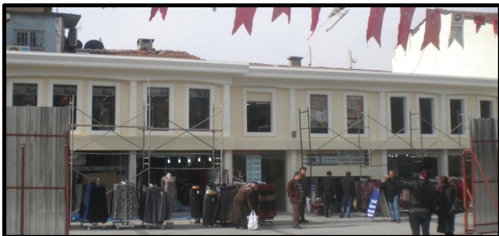
Figure 1.9. Facades of Mahmutpaşa district renovated within the Sanitation Project [11]
