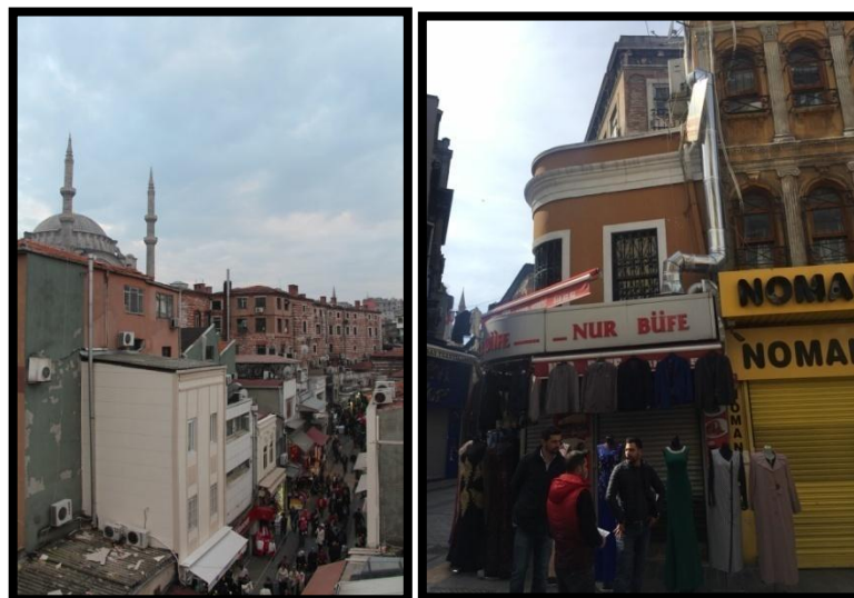
Figure 2.98. and Figure 2.99. Chimneys on facades [13]
