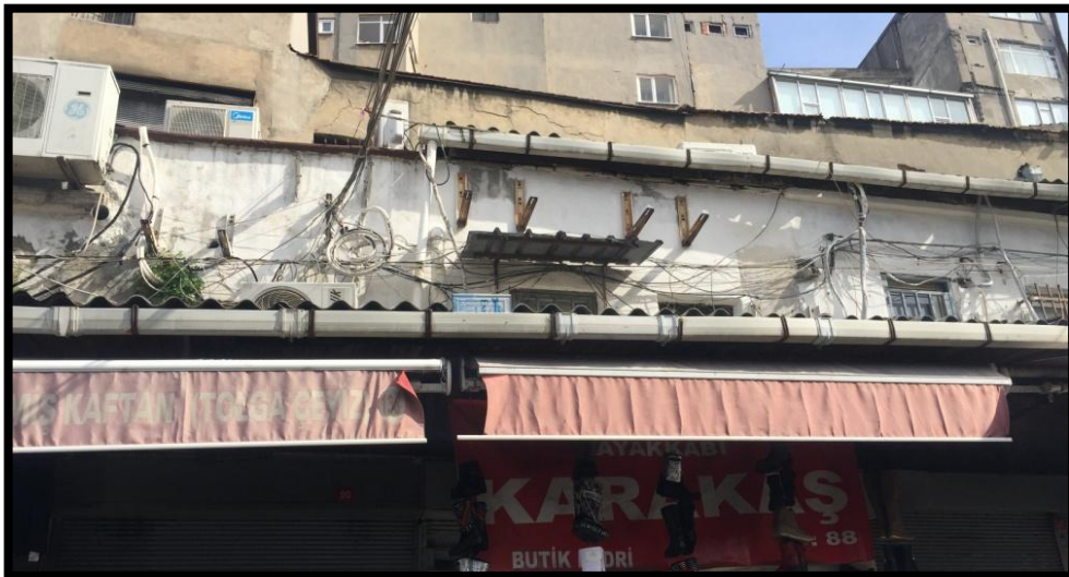
Figure 1.16. Old and unused extensions view [13]
