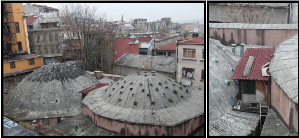
Figure 2.107. and Figure 2.108. Shack-2 view on rooftop of Mahmutpaşa Hamam [13]
