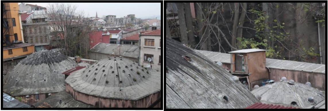
Figure 2.114. and Figure 2.115. Shack-1 view on rooftop of Mahmutpaşa Hamam [13]
