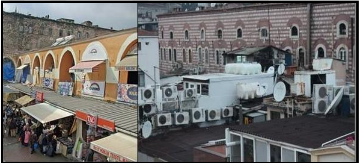
Figure 2.102. Solar panel and its water tanks [13]
