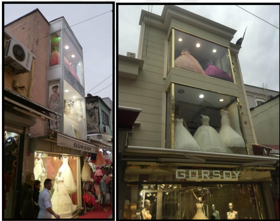
Figure 2.159. and Figure 2.160. Views of facade add-on spaces 3 [13]
