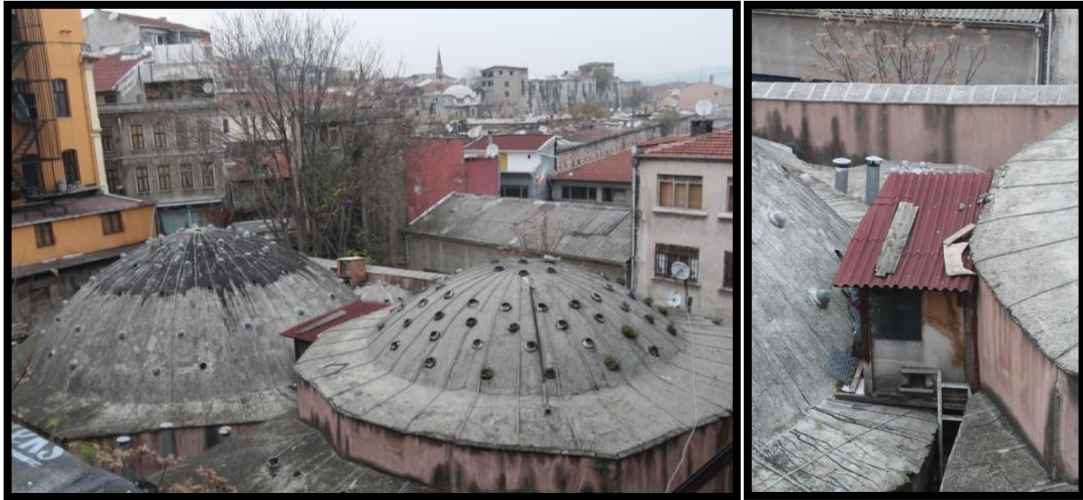
Figure 2.16. and Figure 2.17. Rooftop additions (shack) of Mahmutpaşa Hamam [13]
