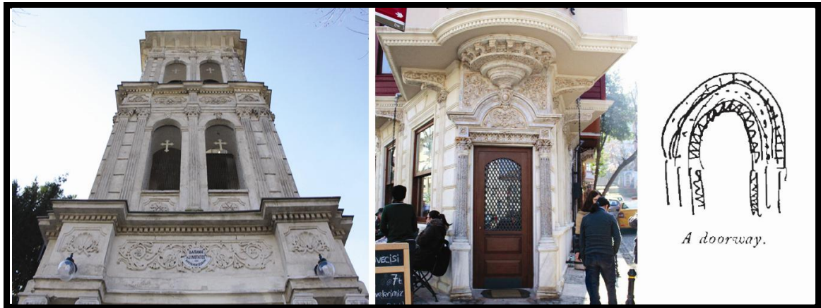
Figure 4.48. Kuzguncuk, İcadiye Street Greek Orthodox Church-Nail Publish House [60][17]
