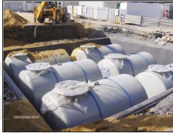
Figure 1.4. Installation of underground petroleum storage tank [8]
