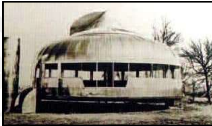
Figure 2.5. Dymaxion House-as its assembly completed: all materials are moved inside the tube on the left side of the photo [14].
