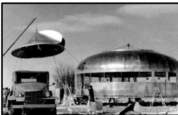
Figure 2.6. Assembly photo, showing the aluminium cladding of the Dymaxion House [14].
