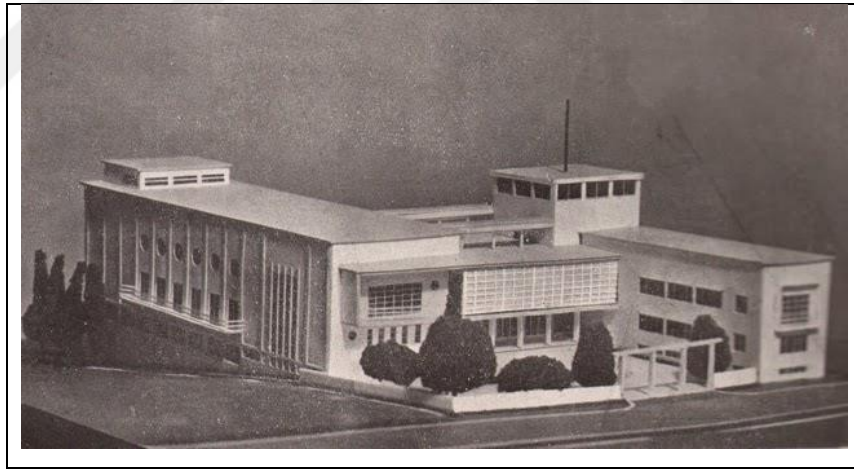
Figure 4.14. Kadıköy Community Center model [96]
