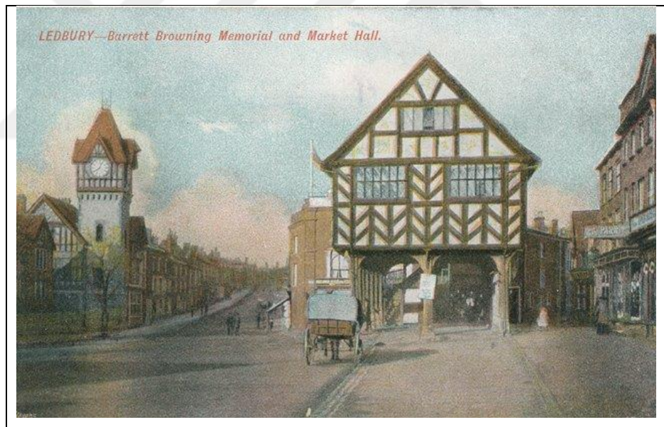
Figure 2.37. A typical two-storey medieval market hall with an open ground floor for trading – Old market hall, Ledbury, Herefordshire, UK, 1617 [50]
