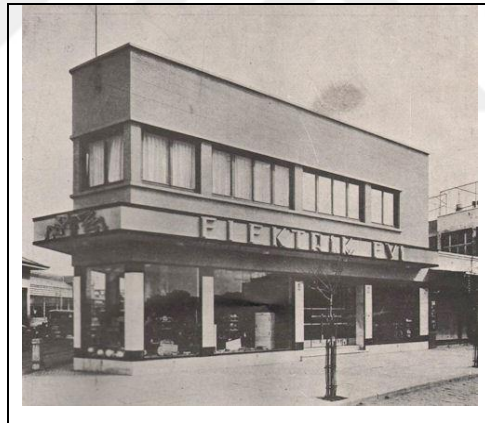
Figure 4.9. Kadıköy Electricity House, Kadıköy, 1928 [95]
