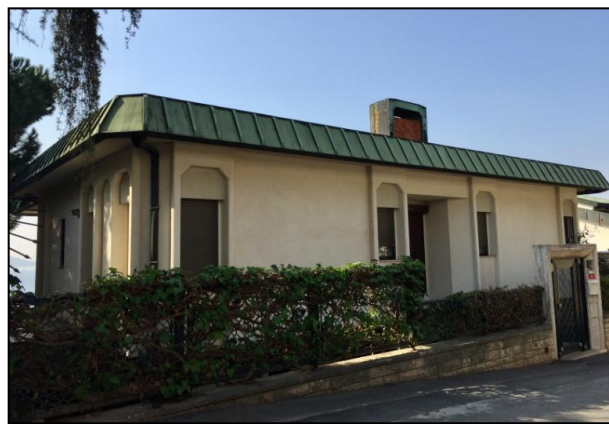
Figure 4.124. Back facade of Orhangazi avenue, no:71 [Photographed by the author, 2018]
