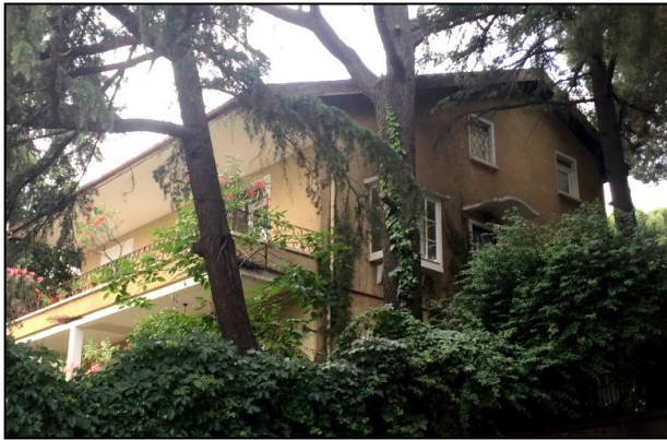
Figure 4.97. Left facade appearance of amlı street, no:62 [Photographed by the author, 2018] (f)
