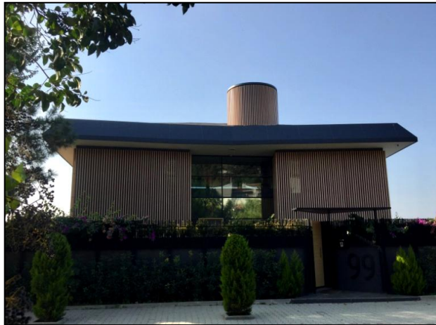
Figure 4.132. Orhangazi avenue, no:99 [Photographed by the author, 2018] (u)
