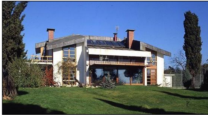
Figure 3.52. Zeytinoğlu house, Ayşe Hayzuran Hasol and Doğan Hasol (1986, Çamlıca) [91]
