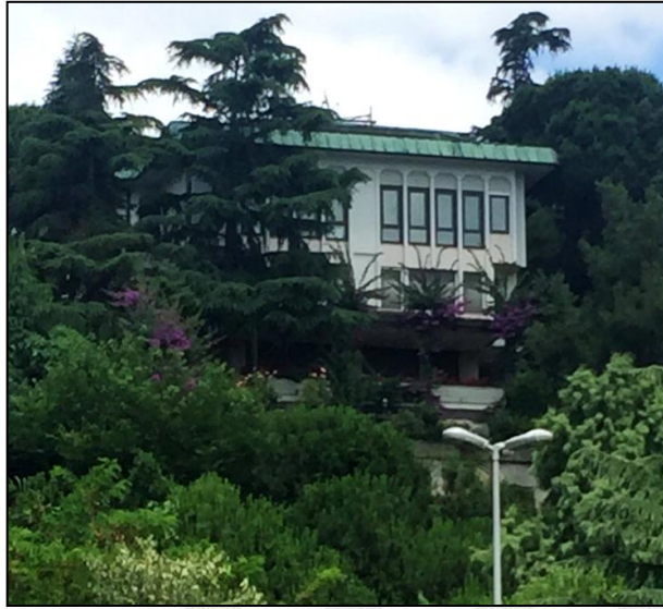
Figure 4.123. Orhangazi avenue, no:71 [Photographed by the author, 2018] (r)
