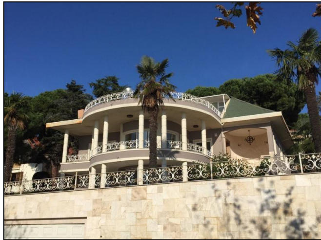
Figure 4.88. Orhangazi avenue, no:38 [Photographed by the author, 2018] (d)
