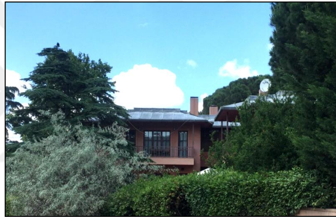
Figure 4.113. Current situation of Zümrüt Akkoyunlu villas [Photographed by the author, 2018] (m)
