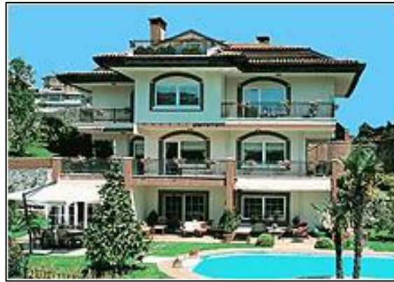
Figure 3.69. Acarkent villas - c type villa (1990s, Beykoz) [96]
