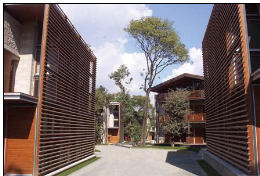
Figure 3.79. Appearance of NP12 houses, 2003 [101]
