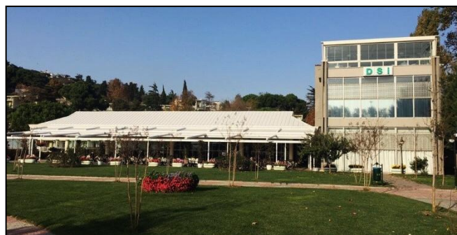
Figure 4.62. DSI restaurant and seminar building, 2018 [Photographed by the author, 2018]
