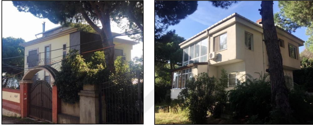
Figure 4.79. Mutlu houses [Photographed by the author, 2018]
