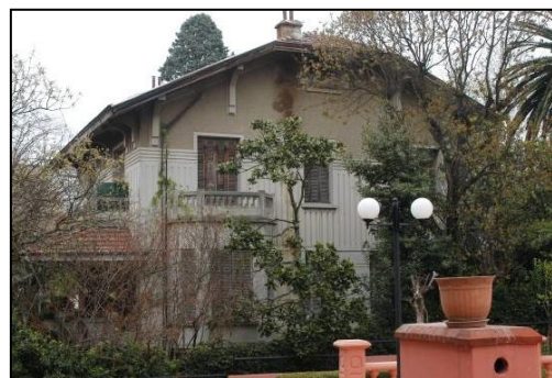
Figure 3.13. Side appearance of Dikmen house [65]
