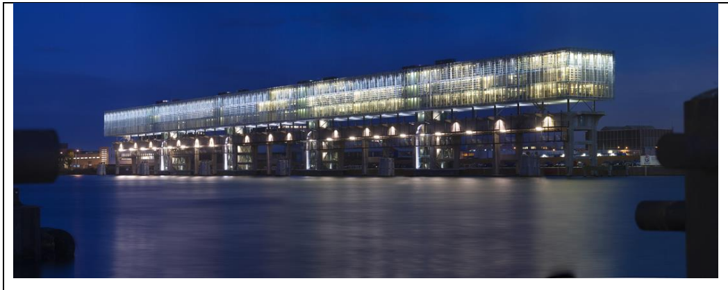
Figure 4.66. View of the Kraanspoor office building giving the impression of floating on the crane way [61].
