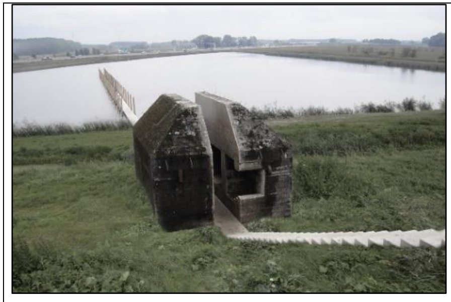
Figure 4.77. The bunker 599 cut through and the wooden path leading to a flooded area [66]
