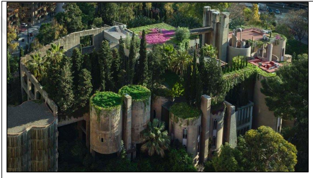
Figure 4.5. Perspective view showing plants climbing walls and hanging from roofs of blocks of La Fabrica [51]
