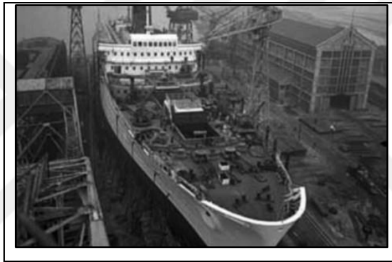
Figure 4.83. Prefabrication of a boat at the AP2 Workshop [67].
