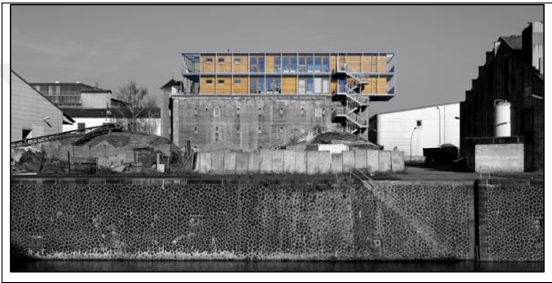
Figure 4.38. View of the bunker [56]
