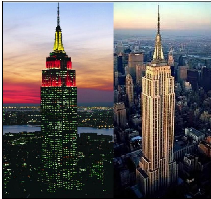
Figure 2.12. The Empire State building, New York, 1929-31 [26].
