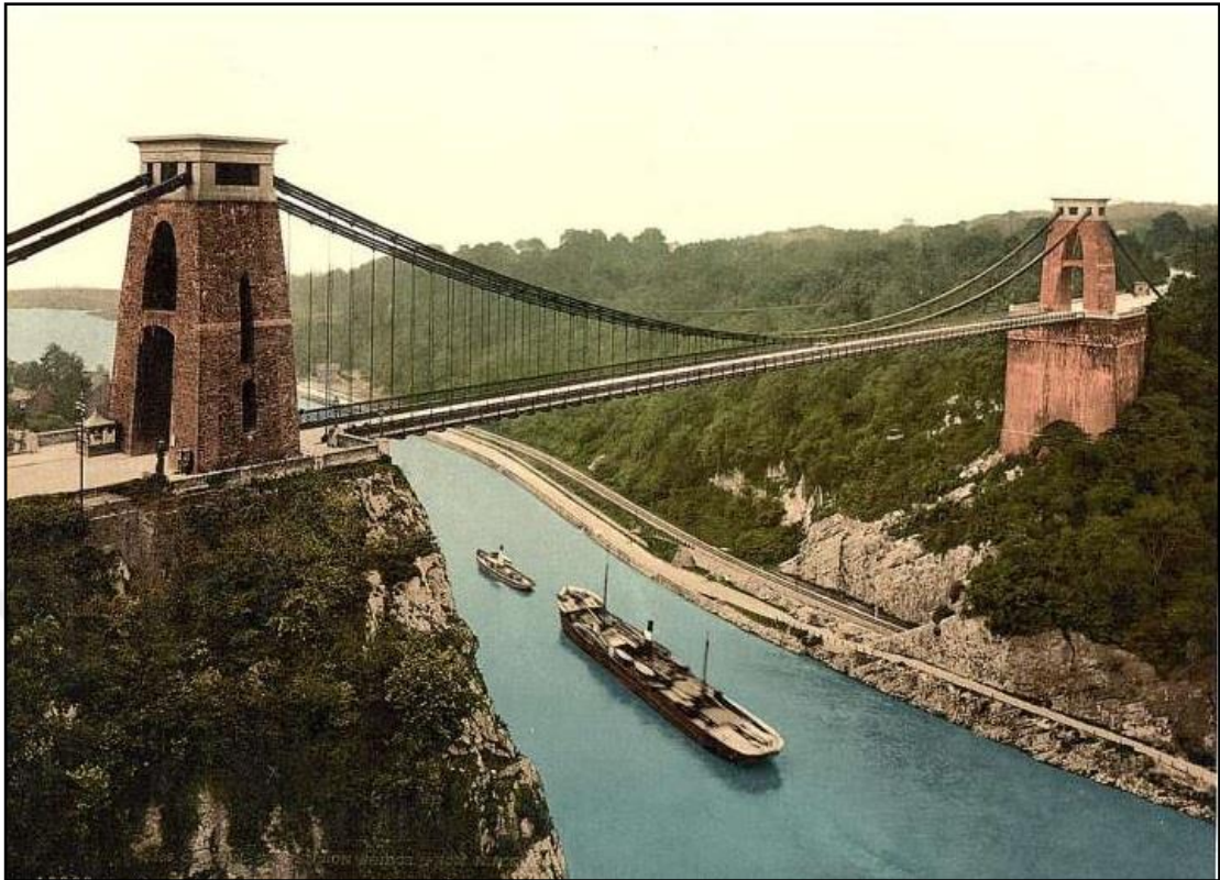
Figure 2.7. Clifton Bridge, England, 1836 [28]
