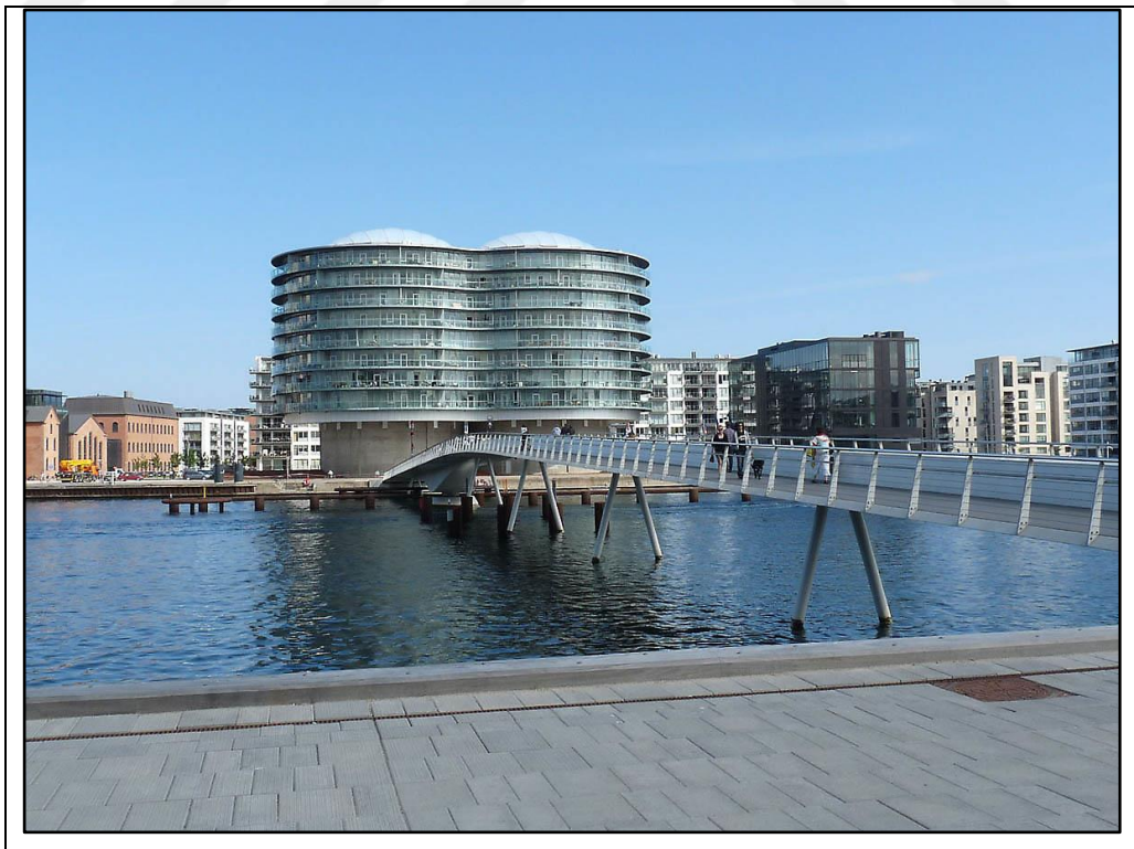
Figure 4.46. The Frøsilø with the Bryggebroen footbridge, connecting both sides of the Bryggebroen island [57]
