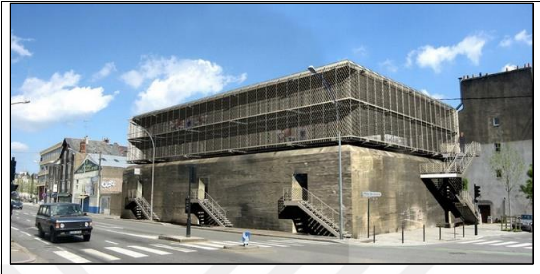
Figure 4.39. View of the bunker [56]
