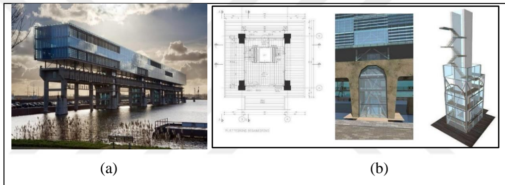
Figure 4.69. (a) View of the Kraaspoor showing the four lifts, (b) detail of the panorama lift [61], [62]
