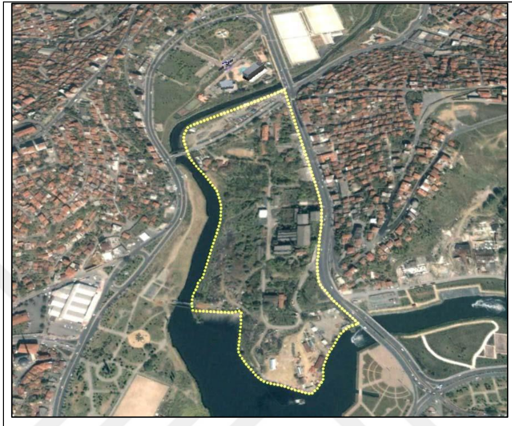
Figure 4.48. Google map of the Silahtaraga Power Plant, 2001
