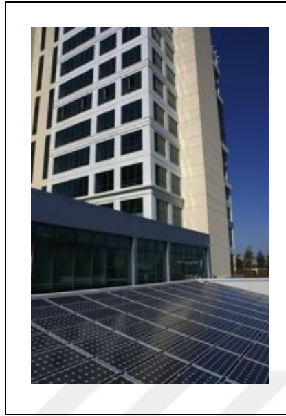
Figure 4.2. The solar panels on the facade of the Anel Building.
