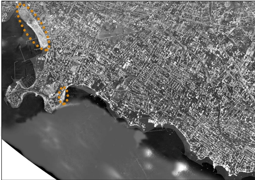
Figure 2.22. Change of Fenerbahçe, Caddebostan, Suadiye and Bostancı coasts with satellite images of 1982 [63].
