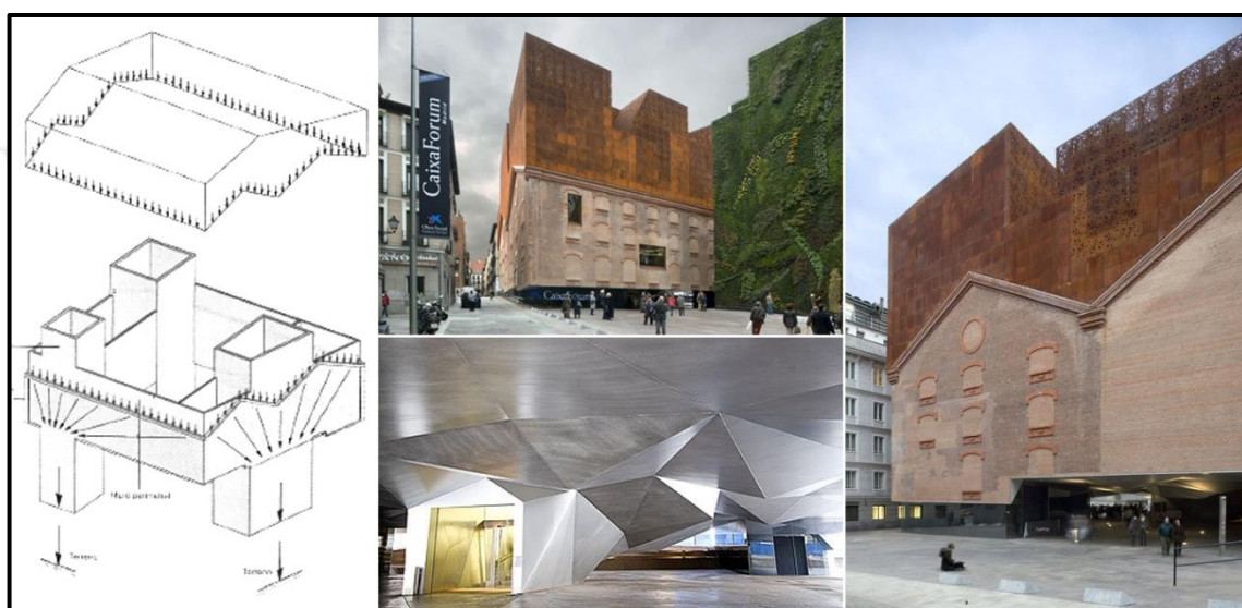
Figure 4.64. New design is supported by three main pillar, which also creates a semi-open space following the main square [257, 259]
