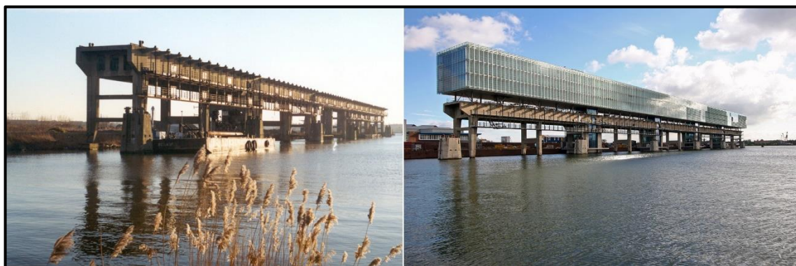
Figure 4.52. Kraanspoor Office Building, before and after its transformation [247]
