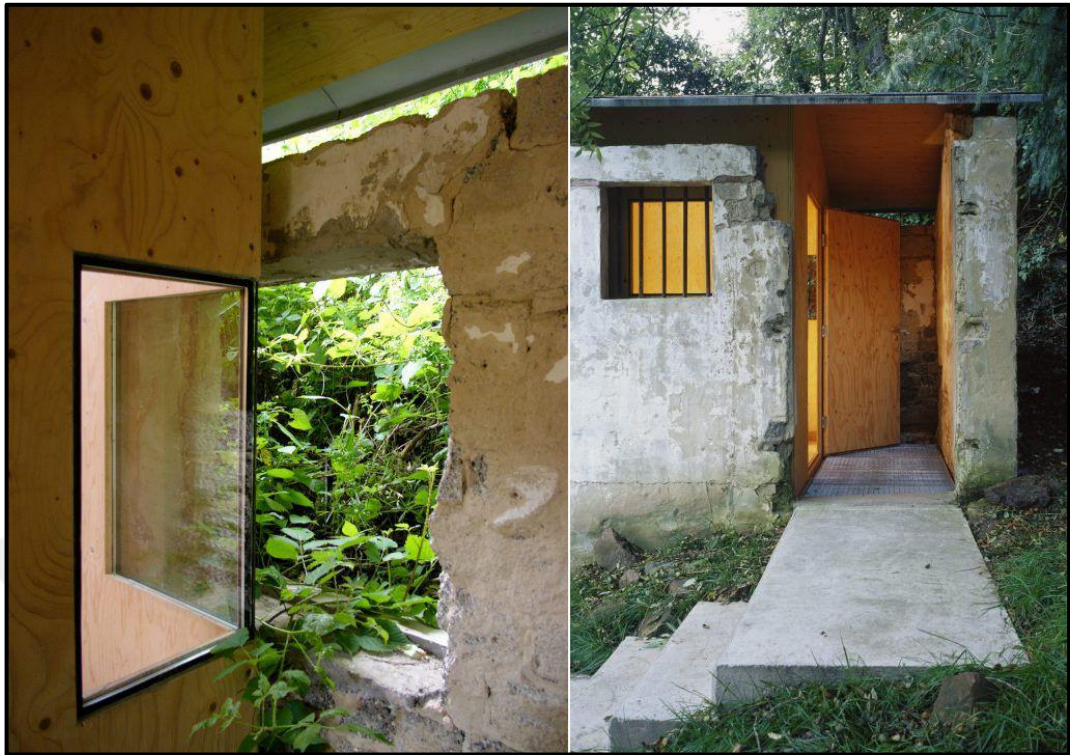
Figure 4.43. Inside volume constructed from Kerto lumber, S(ch)austall, Naumann Architektur, 2005 [229]
