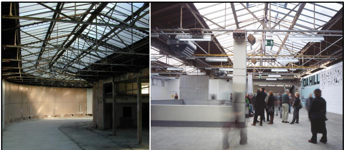
Figure 4.26. During and after the intervention on Palais de Tokyo, first phase, 2002 [211]
