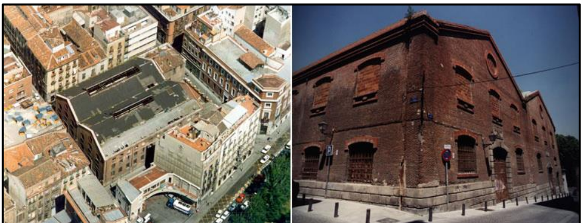
Figure 4.60. Aerial and exterior view of Central Electrica del Mediodia, before transformation [257]
