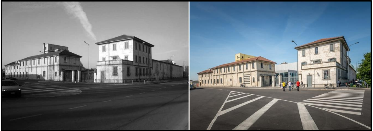
Figure 4.112. Prada Foundation, before and after its transformation [299, 300]
