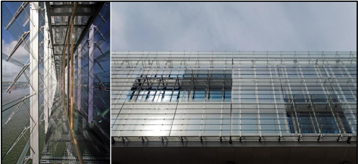
Figure 4.57 Double-skinned façade, Kraanspoor, OTH Architecten, 2007 [247]
