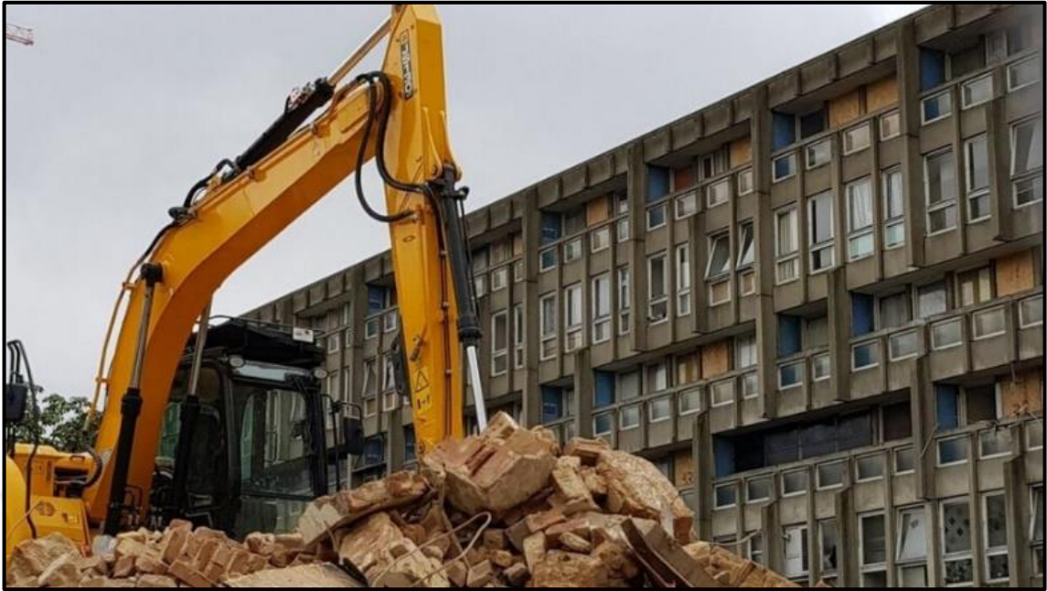
Figure 3.35. Robin Hood Gardens got demolished in 2017 [192]
