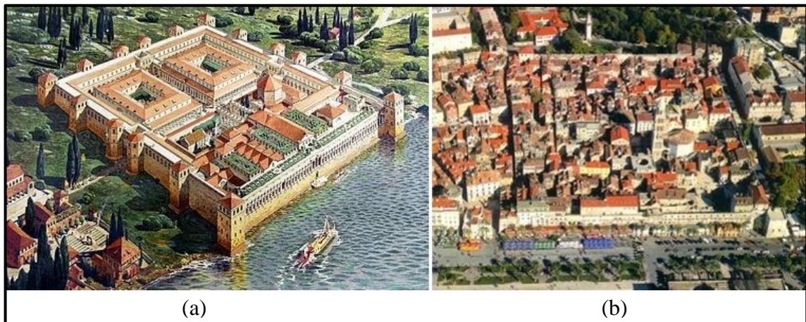
Figure 2.2. Diocletian's Palace in Split, Croatia. (a) Reconstruction, 305 AD [7], (b) Current aerial view [8]
