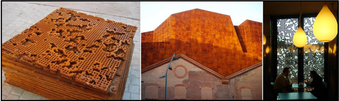
Figure 4.65. Corten steel panels were used on the top extension of CaixaForum Madrid, Herzog & de Meuron, 2008 [257]
