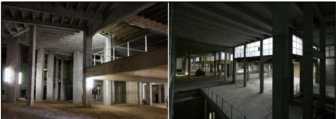
Figure 4.29. Construction of Palais de Tokyo, second phase, 2011 [211]
