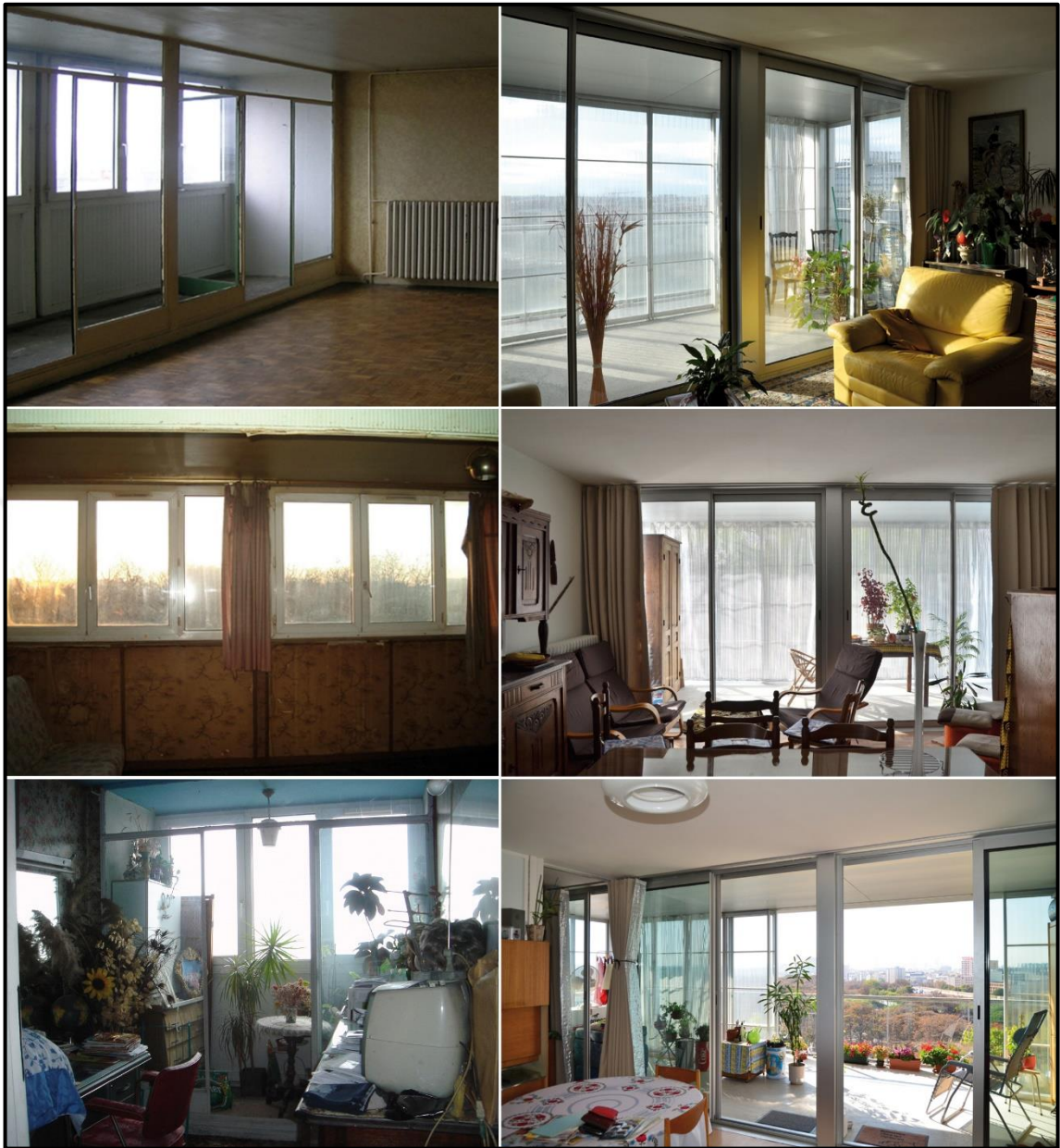
Figure 4.105. Interior views from before (left) and after (right) the transformation, Tour Bois le Prêtre, Lacaton & Vassal, 2011 [290]
