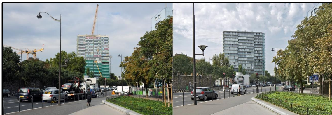
Figure 4.104. Façade views during and after the transformation, Tour Bois le Prêtre, Lacaton & Vassal, 2011 [290]
