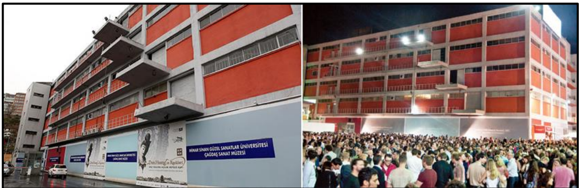
Figure 4.125. Warehouse number five, before transformation [316, 317]
