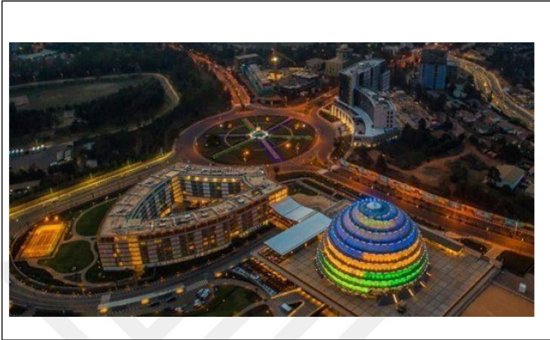
Figure 3.22. Sky view of the immediate surrounding of the Kigali Heights [125]
