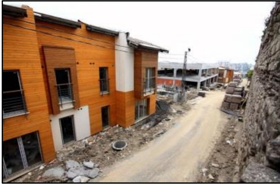
Figure 2.5. New housing in the neighborhood [29]
