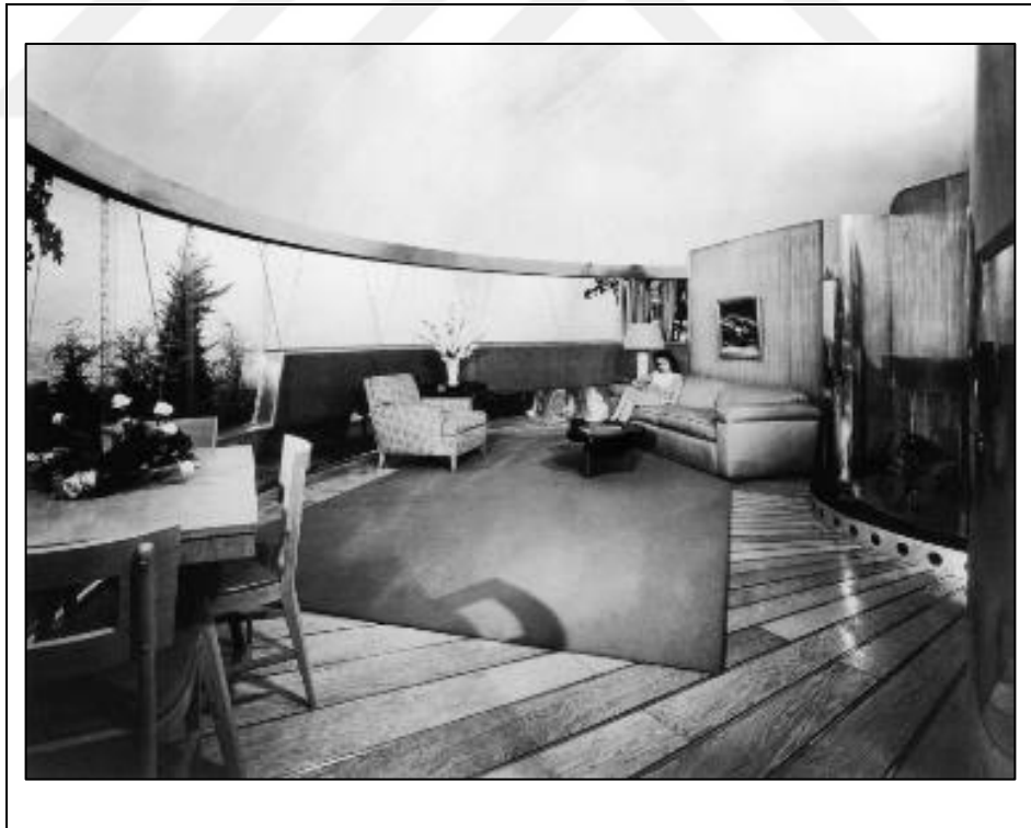
Figure 2.17. Interior of Dymaxion House, Wichita (1946) [50].
