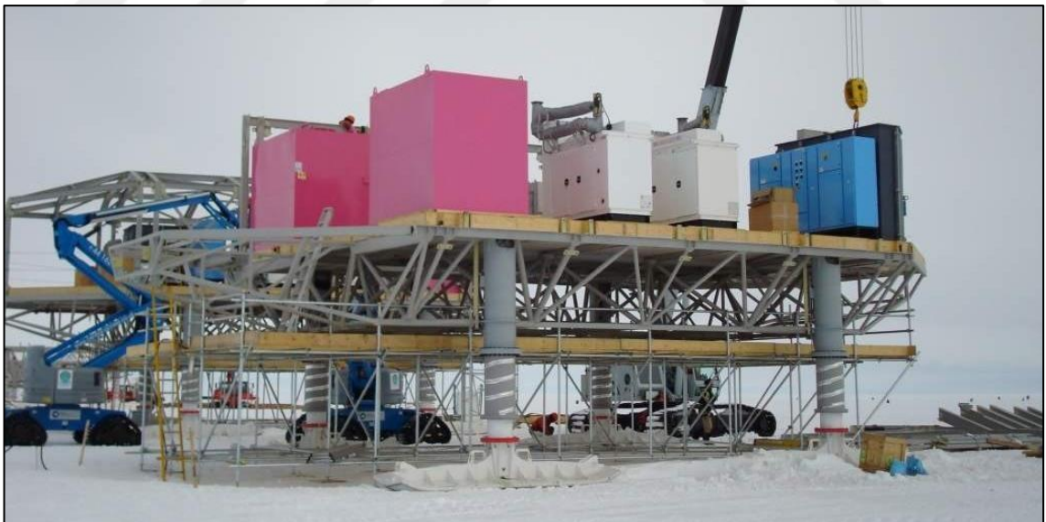
Figure 2.37. Image of VI Halley Research Station under construction [66].
