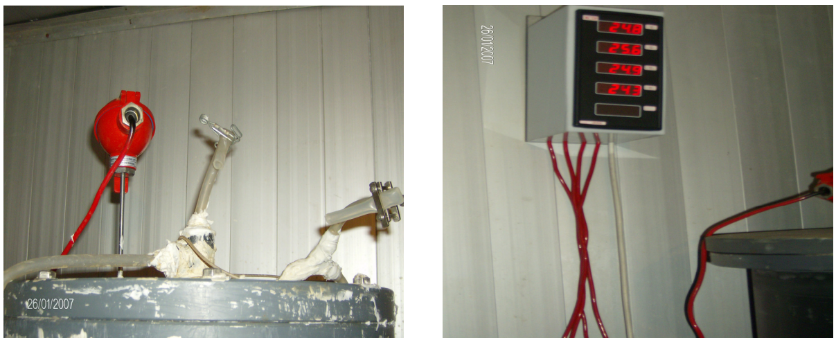
Figure 4.5. Thermocouple and temperature reading
