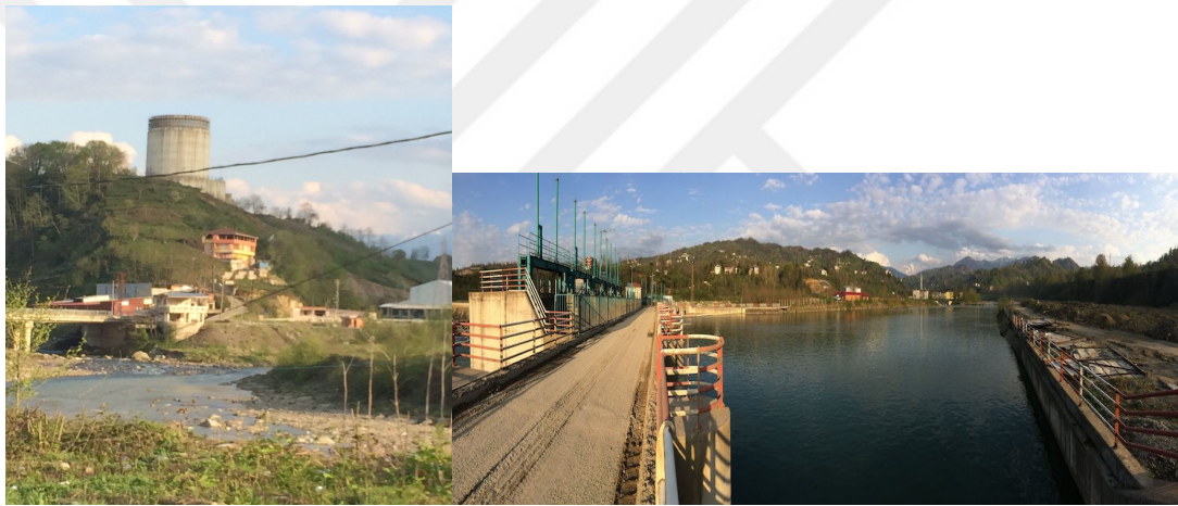
Figure 7.5. The photo on the left shows the surge tank of the İncirli HES . The photo on the right is taken from the corner of the artificial pool behind the water-intake facility that was constructed on the riverbed for the İncirli HES (Photos by the author).
