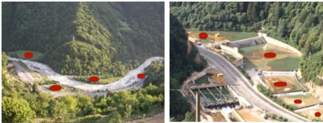
Figure 6.3. The sedimentation deposit sites (red spots) before the construction of the water-intake facility of the Cevizlik HES and after. Source: Photo on the left by Osman Coşkun. Photo on the right by the author.
