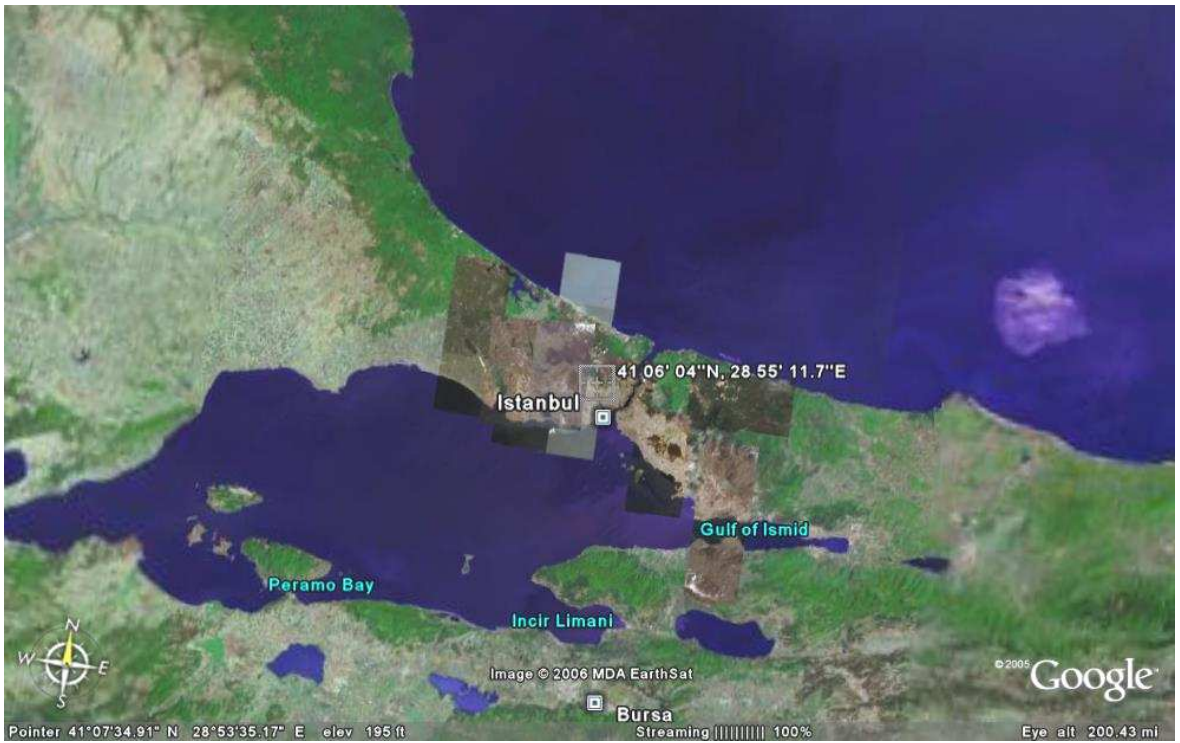
Figure 2 - 1: Satellite view of Alibey Earth Dam. Courtesy of Google Incorporation. Google Earth Virtual Globe Software, 2006.
