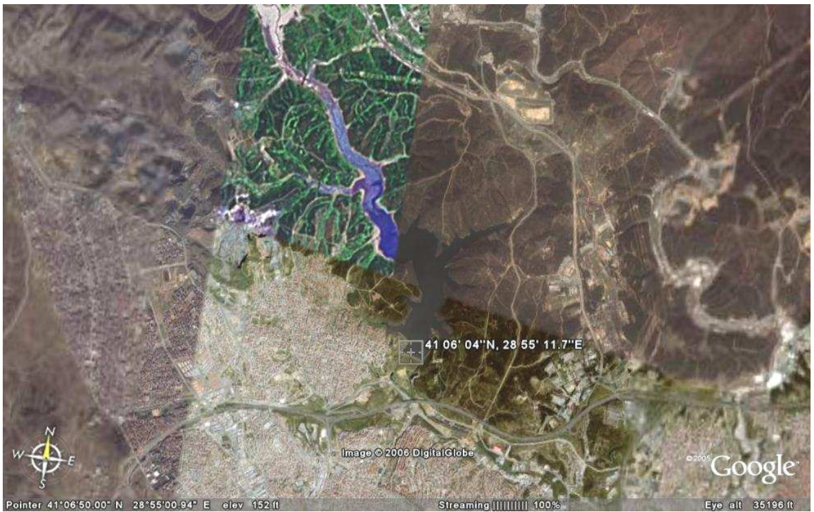
Figure 2 - 2: Satellite view of Alibey Earth Dam. Courtesy of Google Incorporation. Google Earth Virtual Globe Software, 2006.
