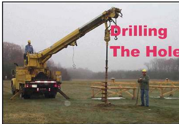
Figure 3.14. Drilling the hole for soft ground concrete pillars
