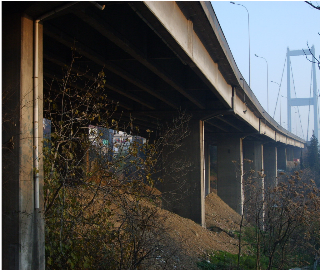
Figure 3.1. Side view picture of Ortakoy V409 Viaduct
