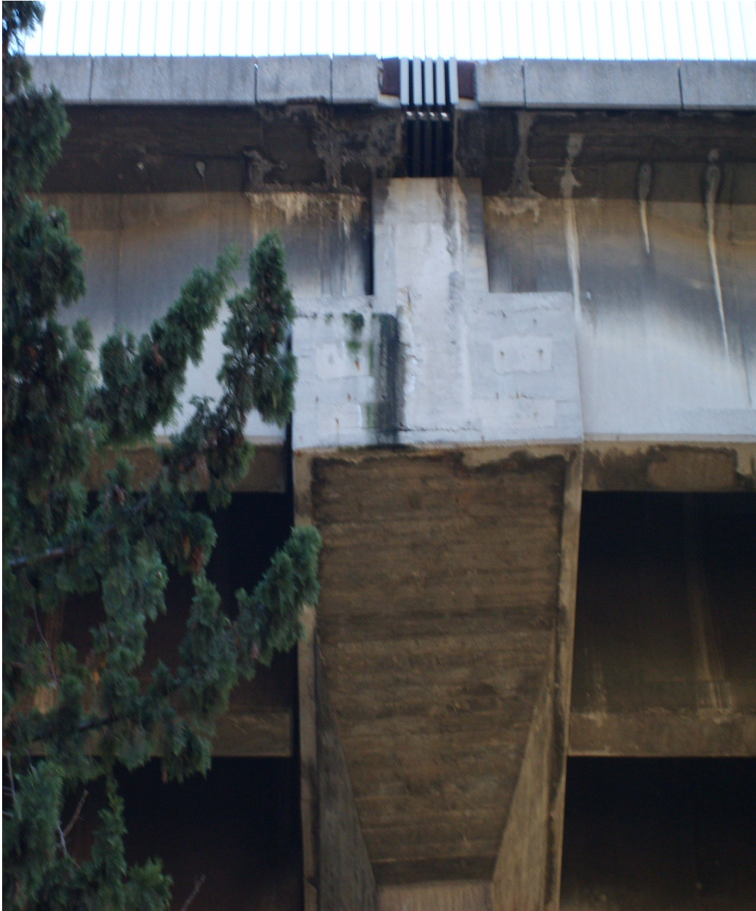
Figure 3.9. Expansion joint at pier 4
