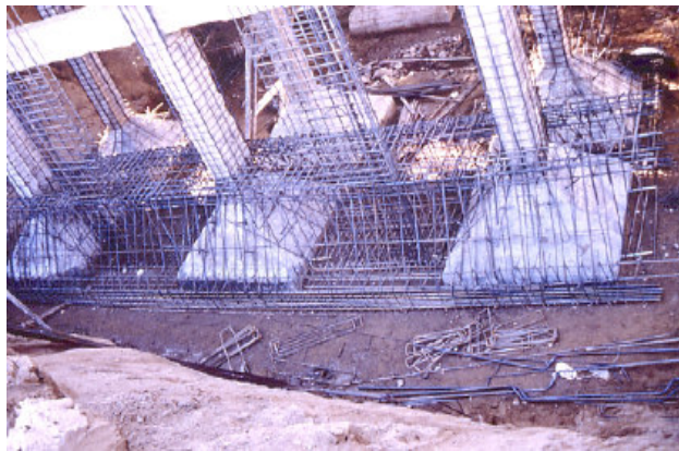
Figure 1.8. Reinforced concrete jacketing in-situ view
