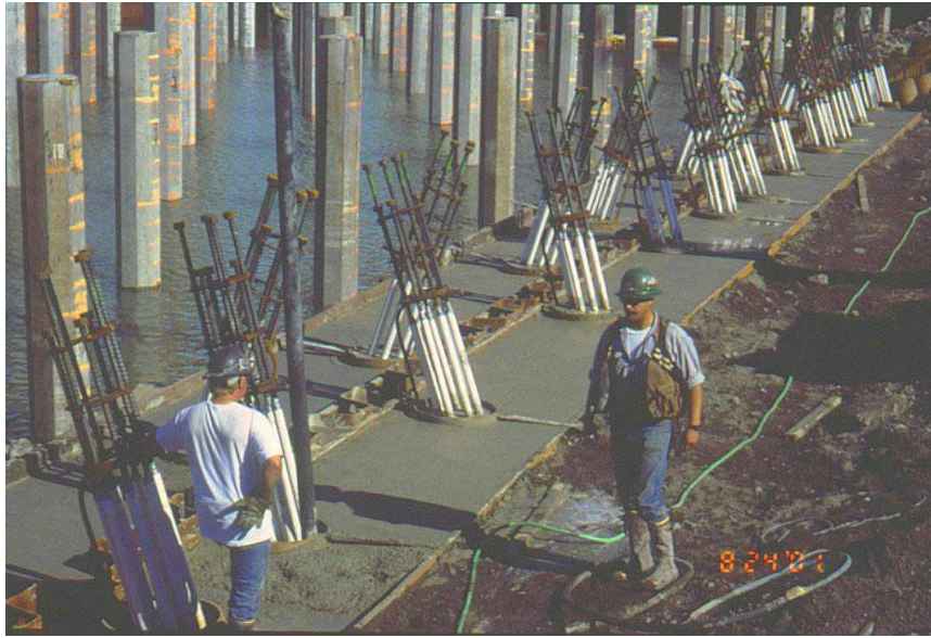
Figure 6.7. Pipe piles with a tension fuse detail under construction (Harn, 2004)
