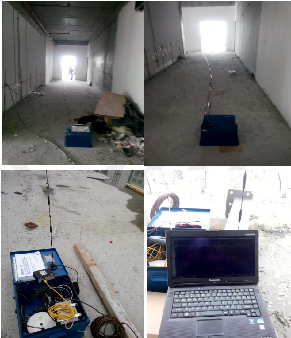
Figure 4.4. Experimental set-up located on the first basement, 7 th and 15 th story (Case 2)
