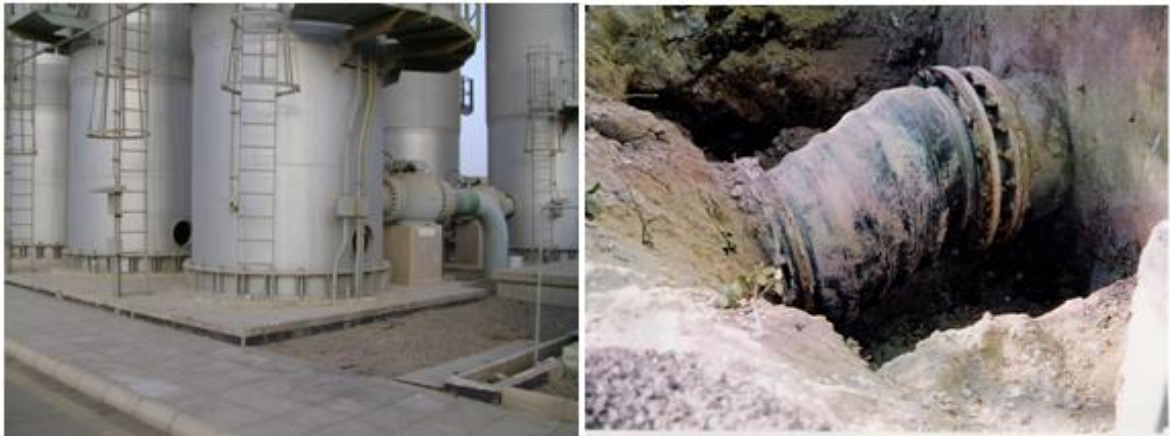
Figure 1.6. Flexible pipe connection and typical deformation.
