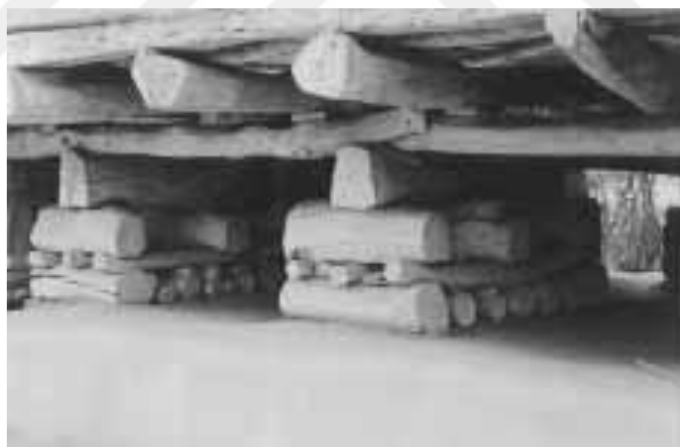
Figure 2.2. Use of Timber as Base Isolator (Hussain, 2014).
