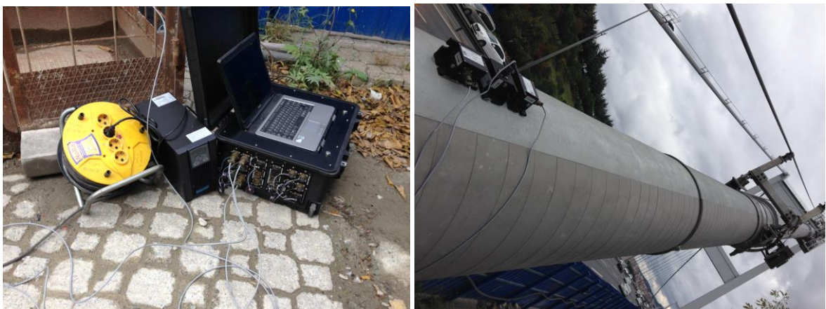
Figure 2.8. Temporary seismic network installation for back-stay cable (strong motion accelerometer, transducer, power supply and laptop computer).
