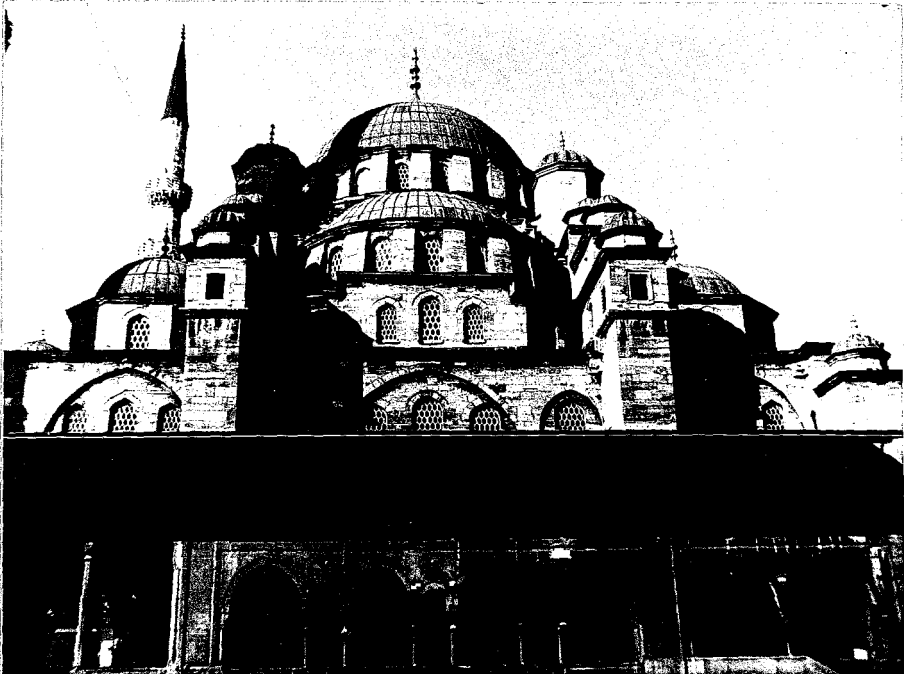
30. Yeni Cami. View of covering system from west façade.
