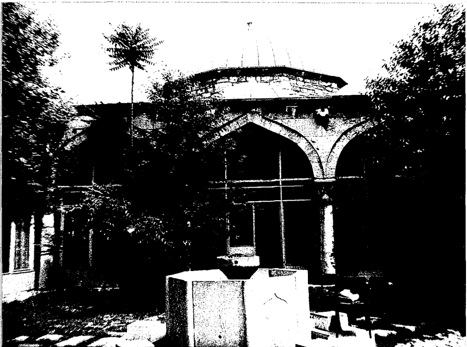
74. Bayram Paşa Complex. Medrese courtyard.
