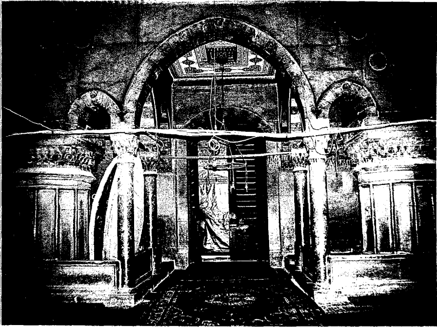
35. Yeni Cami. Interior view of western façade.
