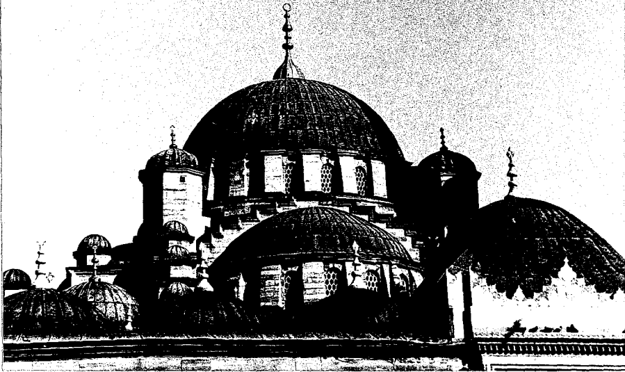
31. Yeni Cami. View of covering system from north façade.
