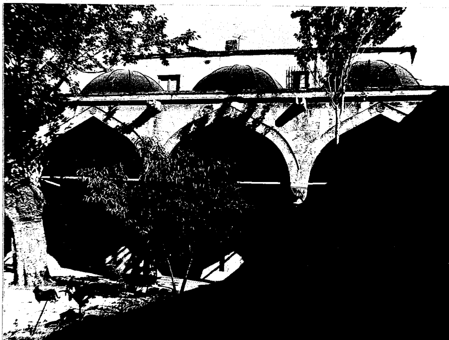
65. Ekmekçioğlu Ahmet Paşa Complex. Arcade in the medrese courtyard.
