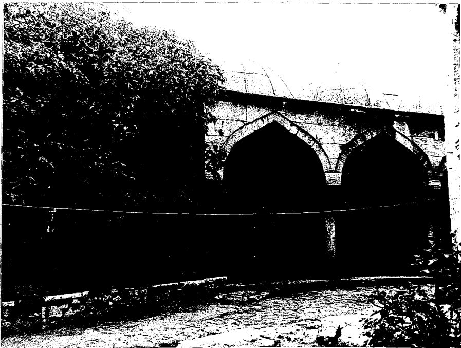
70. Bayram Paşa Complex. Arcades of the tekke cells ( cemetery -hazire- on the left )
