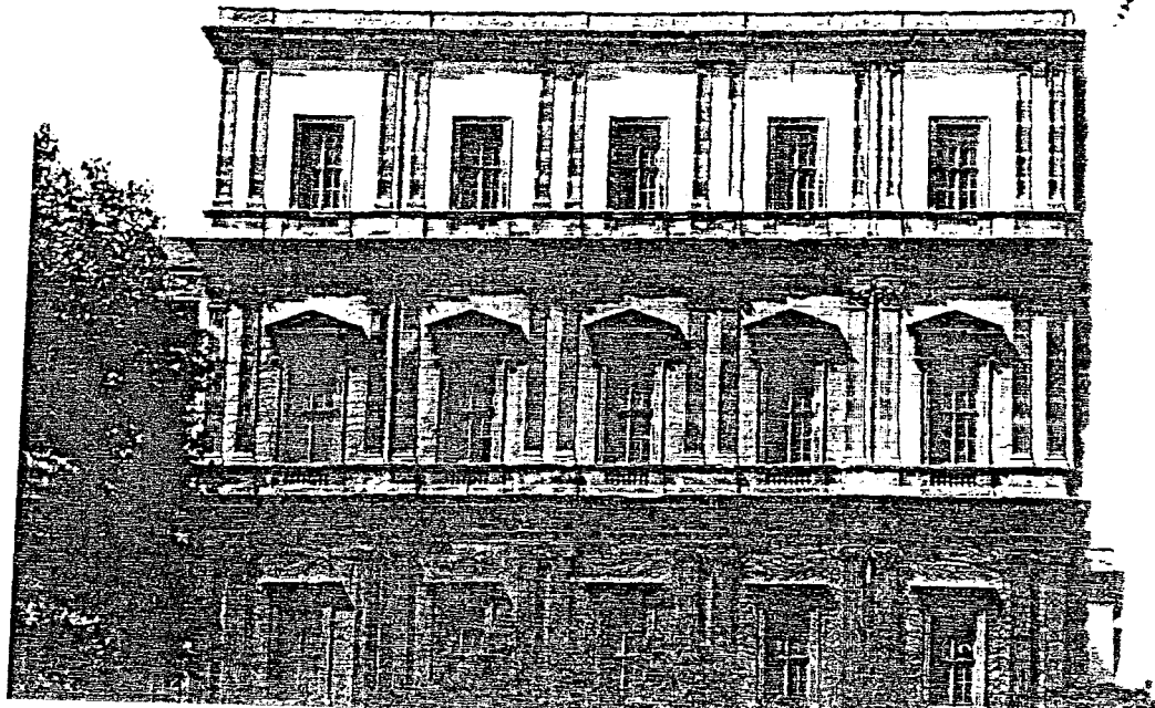
Fig. 8 View from South
