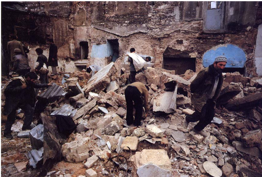
Figure 13. Ara Güler, 'Pillagers who came to collect pieces of wood and iron right after the demolitions in Eminönü. Eminönü', 1986
